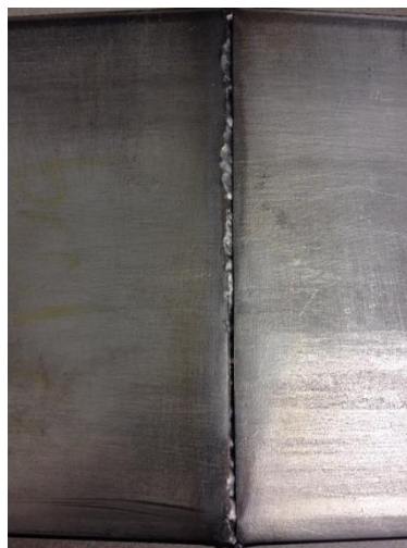
Figure 6.10 Back side of the plate which shows lack of root penetration
