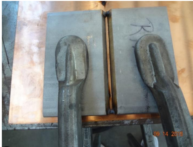
Figure 6.9 copper plate is used to get lack of root penetration
