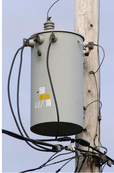
Figure 5. 50 kVA single phase pole mount transformer [17]
