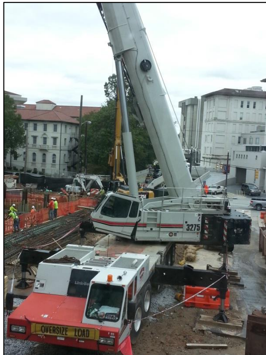
Figure 1: Crane powered by loud hydraulics
