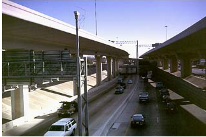
Figure 5.7. Roadway monitoring via video cameras [141]. The use of CRFIDs could allow for the monitoring of larger areas with less maintenance and infrastructure than video monitoring.
