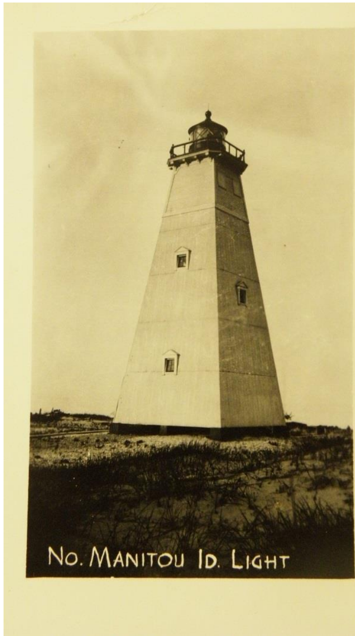
Figure 6. North Manitou Island Light. Bentley Historical Library, Post Card Collection, Box 9, North Manitou.
