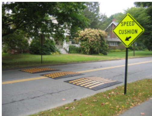
Figure 29 Temporary speed cushions
