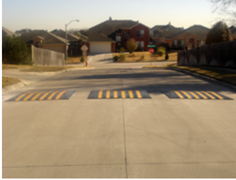
Figure 28 Permanent speed cushions (25)
