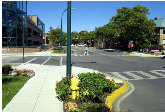
Figure 36 Curb extensions at an intersection (44)
