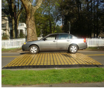
Figure 25 Speed table constructed from rubber (25)
