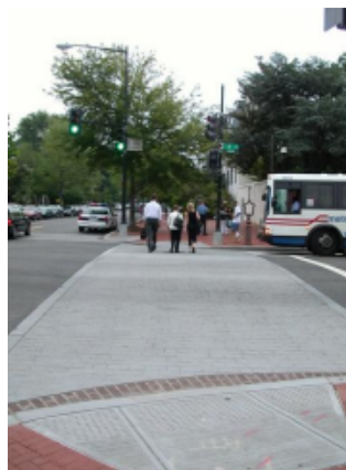
Figure 35 Stamped concrete pedestrian crossing (44)
