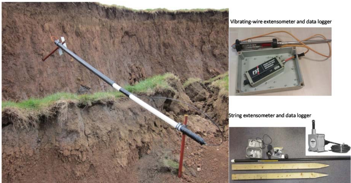
Figure 3.10 Vibrating-wire and string pot extensometer installations, which is parallel to the shear surface.
