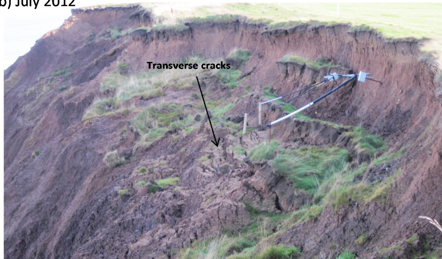
Figure 7.16 The photographs of the progressive landslide development of mudslide: a) the transverse cracks were observed clearly in March 2011 (a) and (b) some cracks have developed to become a part of mudslides during wet period (i.e. July 2012).
