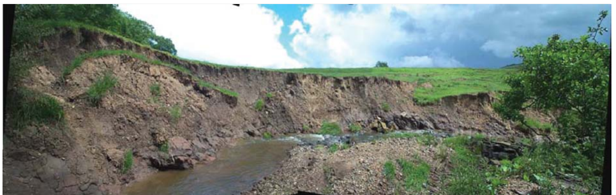
Figure 7.2: The extent of bank erosion along Glaisdale Beck. Source: Jeff Warburton.
