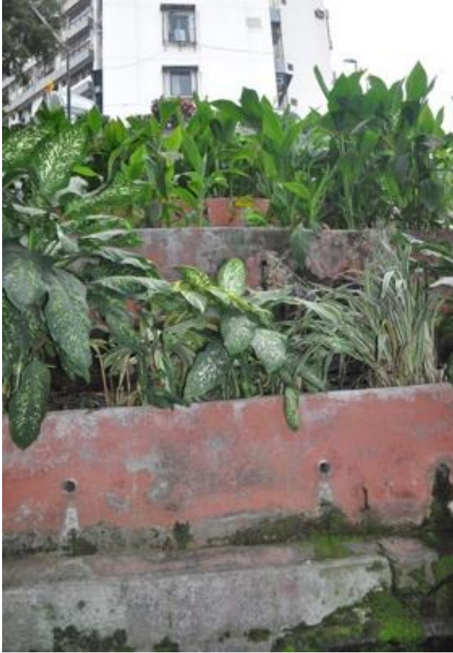
Figure 6.7: Flowerbeds are used to filter water at Kanti Apartments (Source: Author)
