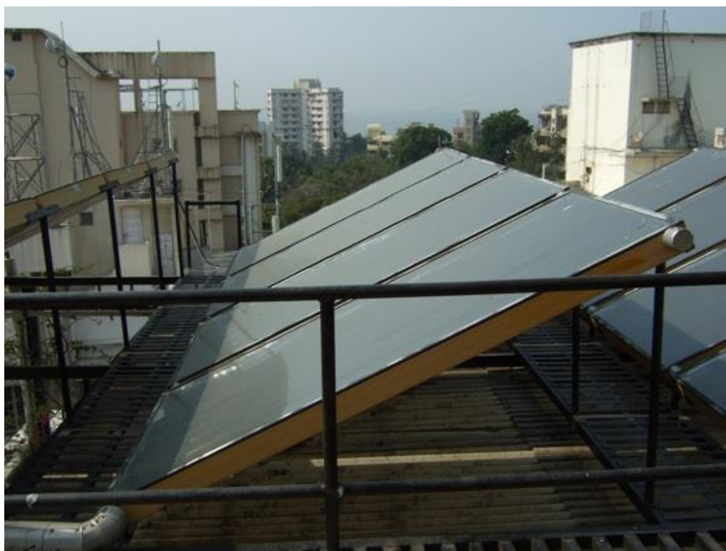
Figure 6.13: Solar water heating was installed after rainwater harvesting in Sealine (Source: Author)
