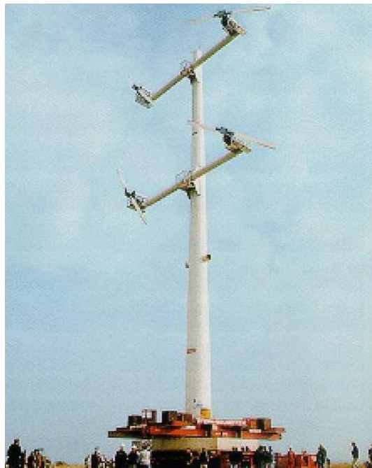
Figure 2.6. A Lagerwey 4 rotor system [9]
