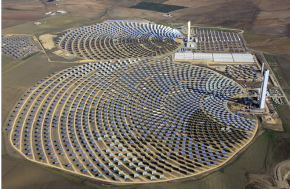
Figure 1 – Abengoa’s solar power towers PS10 (top) and PS20 (bottom) in Seville, Spain. The large field of mirrors reflects sunlight towards the top of the power tower, seen in the right of the image. From Abengoa (2009).
