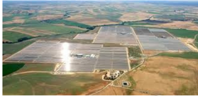
Figure 1.8: Solnova 1 and 3 Parabolic Trough based Solar Thermal Plant (Source: Abengoasolar.com)
