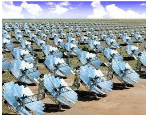
Figure 1.11: Stirling Energy System’s 300 MW commercial solar thermal power plant in California (Source:mtholyoke.edu)
