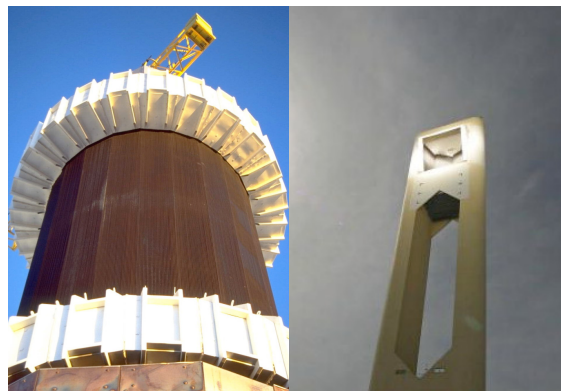
Figure 3.22: Two different configurations for Receiver 1) External Receiver 2) Cavity Receiver (Source: Wagner, 2008)
