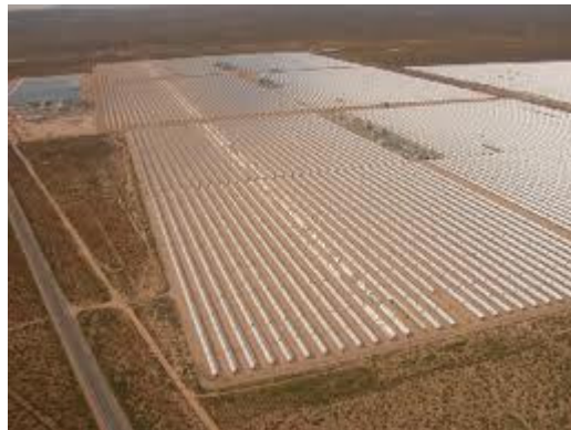
Figure 1.9: SEGS-III (Source: NREL)
