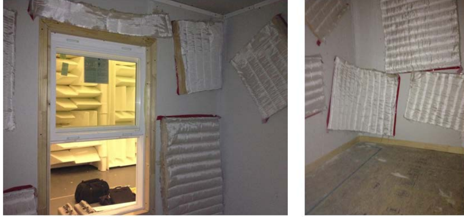
Figure 4.5: Insul-Quilt blankets stapled to test house interior to simulate absorption
