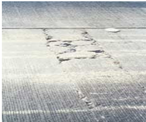
Figure 2.14 High severity punchout [6]
