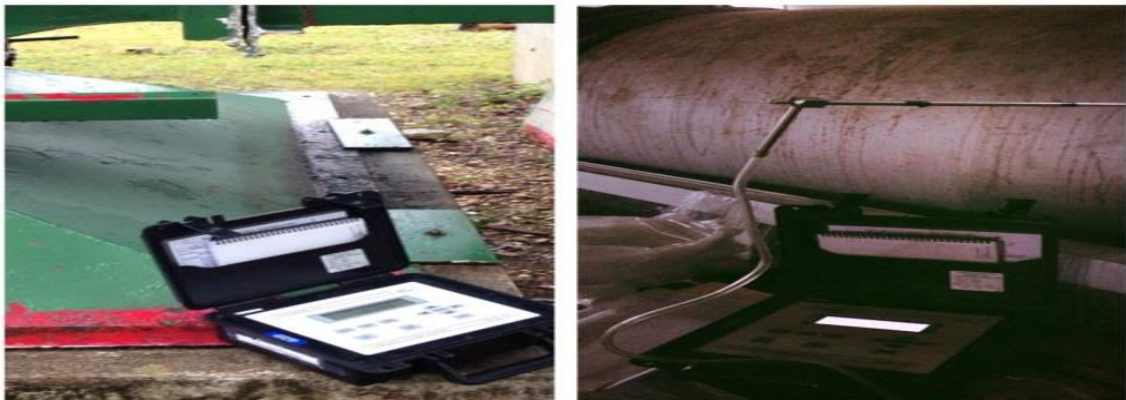
Figure 6.4. Transducers usage through the ducting
