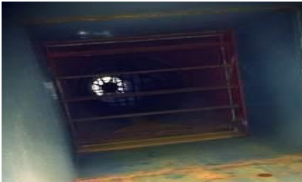
Figure 6.7. Louver blades at 0° angle position
