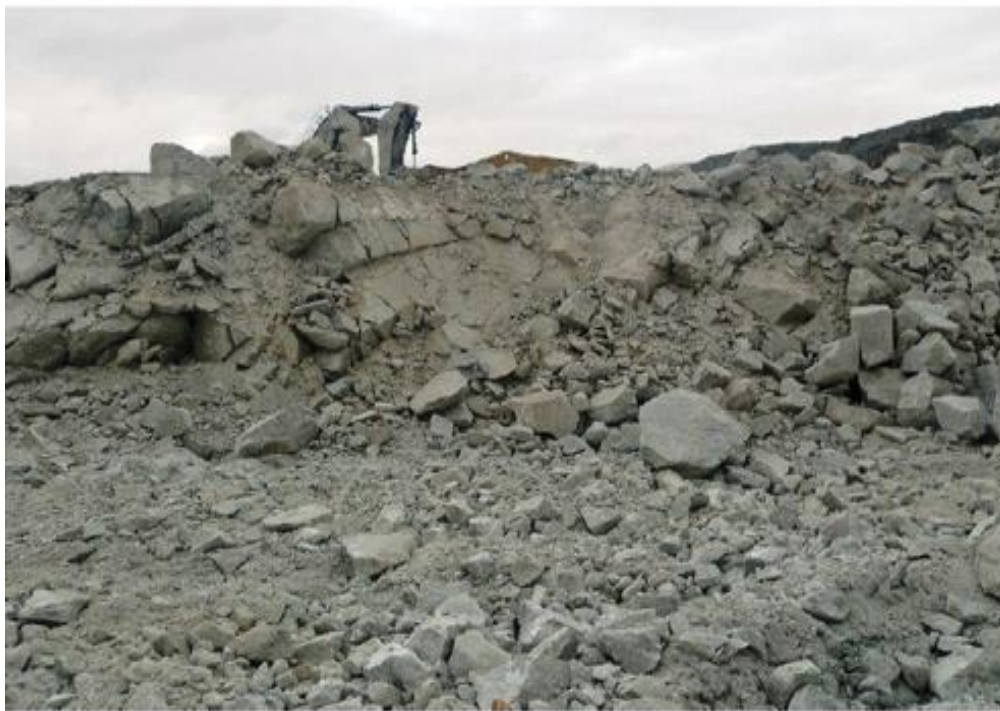
Figure 1.2. Visible rock formation after blasting
