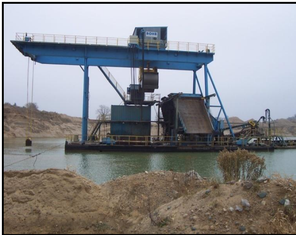
Figure 1.1 Clamshell dredge on site
