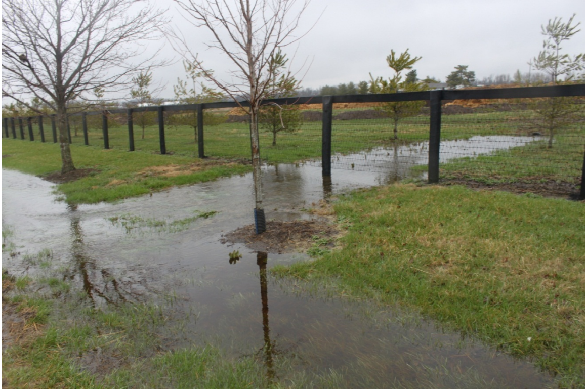
Figure 2.5: Ephemeral Stream Flows through Culvert before Entering Roadside Ditch.
