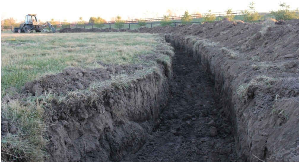
Figure 2.10: Modified contour weep berm excavated trench for woodchip bioreactor with excavated soil positioned on contour weep berm footprint.
