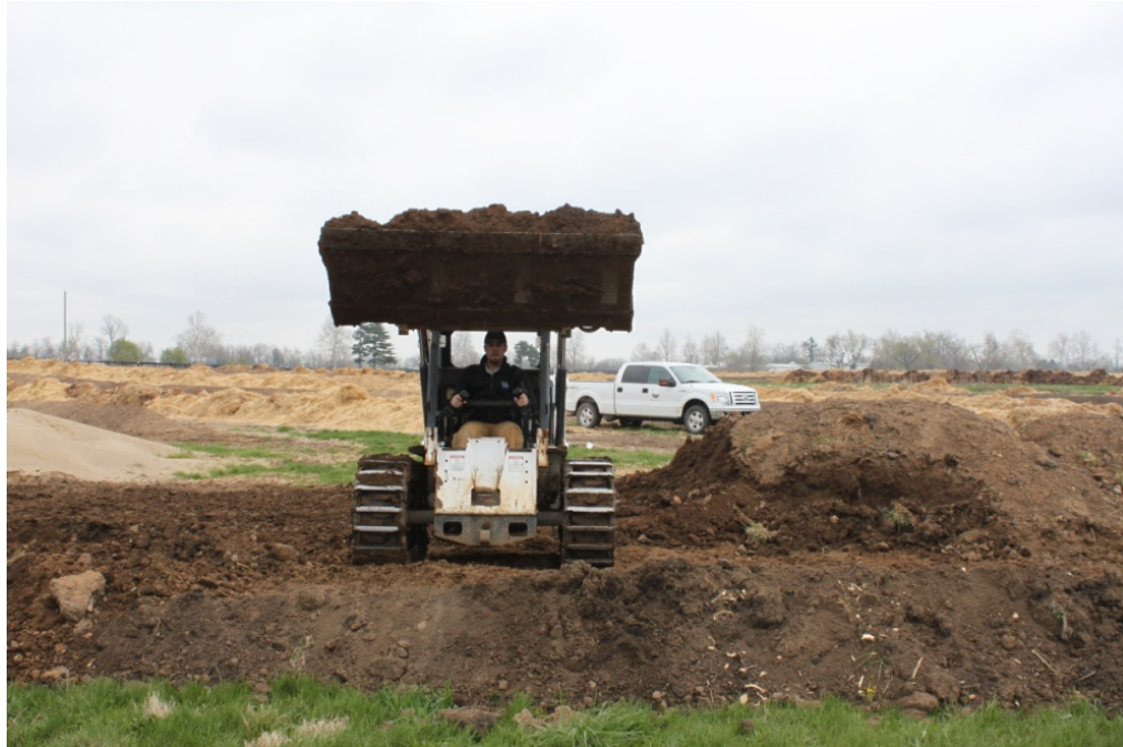
Figure 2.16: Modified contour weep berm construction using a skid steer loader.
