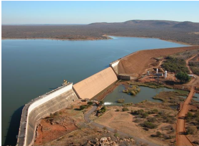
Figure 2.5: Flag Boshielo Dam with outflow into the Olifants River.
