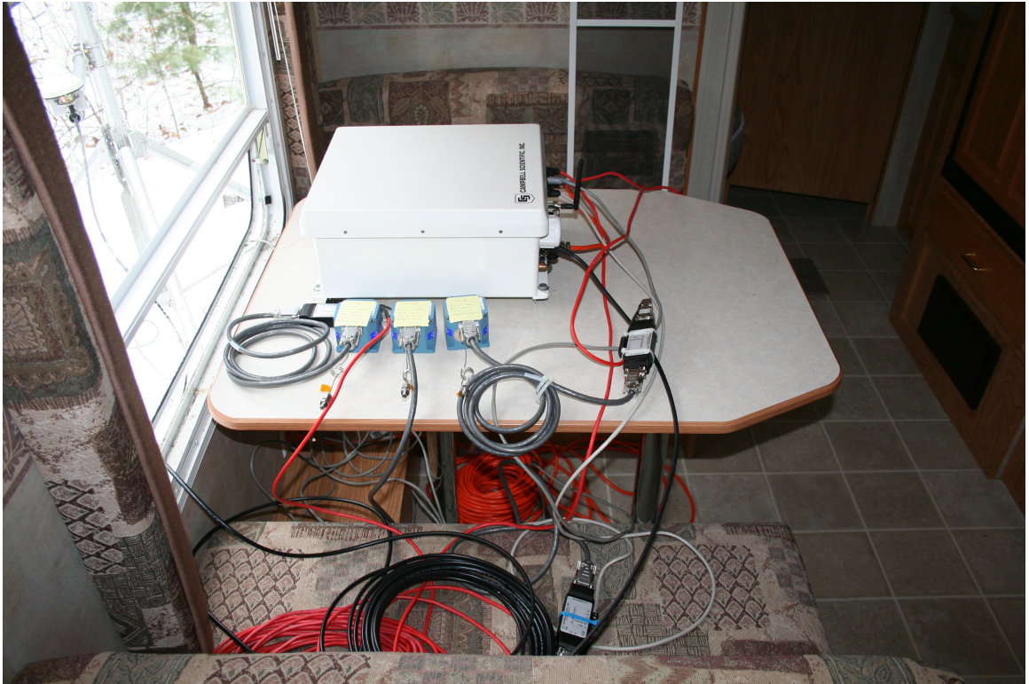
Figure 3.3. Photograph of the barometers with data logger inside the travel trailer: It shows the barometers (cube-like in blue color) with data logger (white colored box) on a table top.
