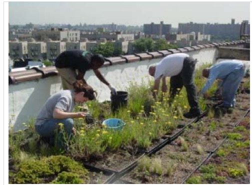
Figure 21: BEST Green Job Training participants install a green roof. Majora Carter Group
