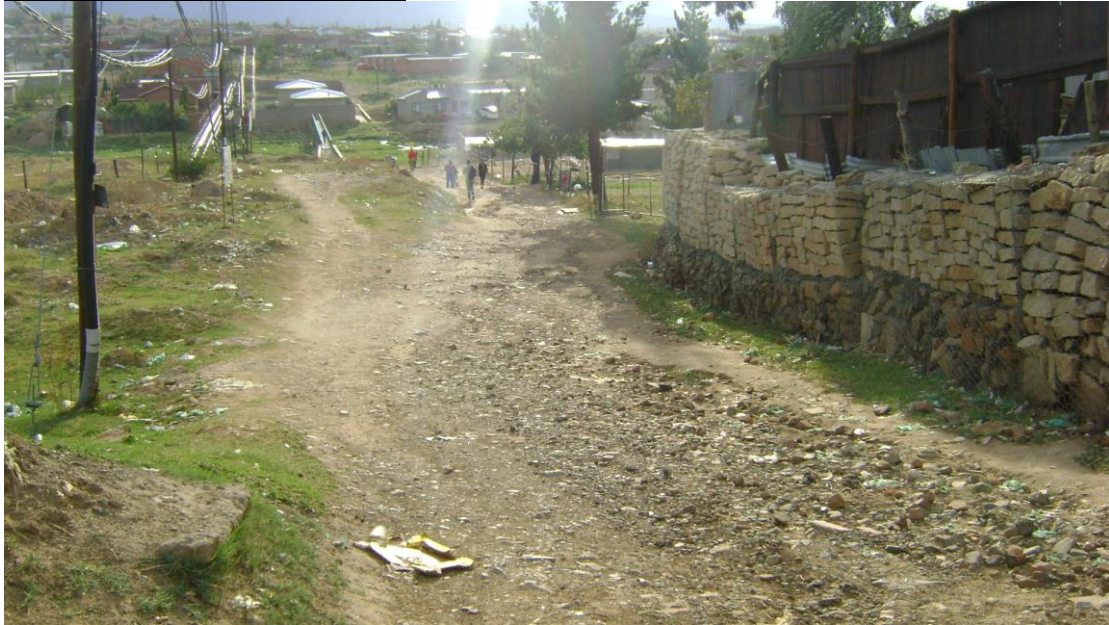
Figure 11: Earth access road
