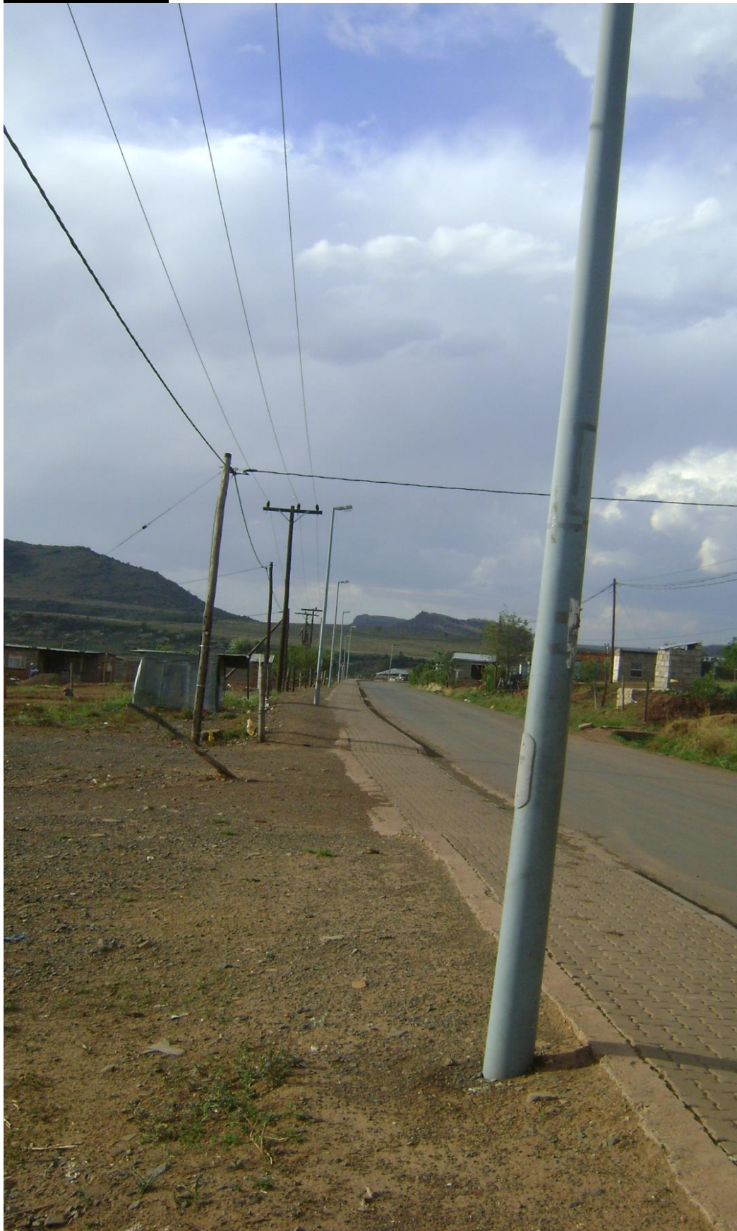
Figure 10: Tarred access road, street lights, and telephone and electricity lines on the pavement
