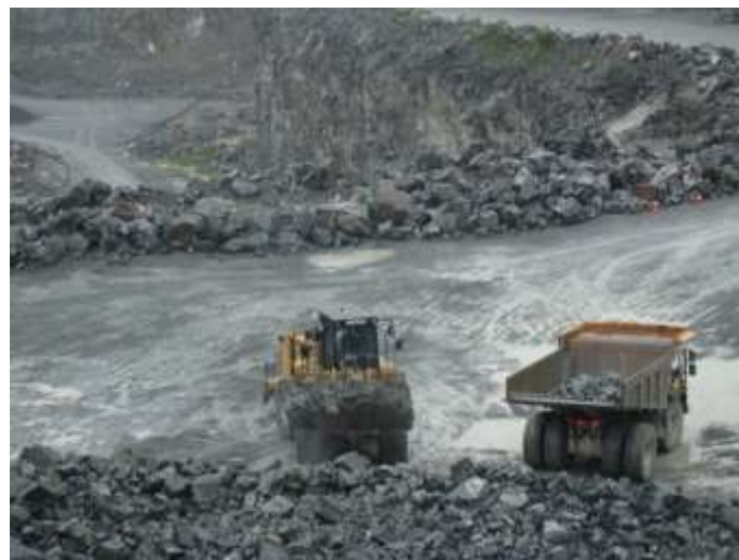
Figure 3.8. Shot Mucking (Catipillar 990 Loader)
