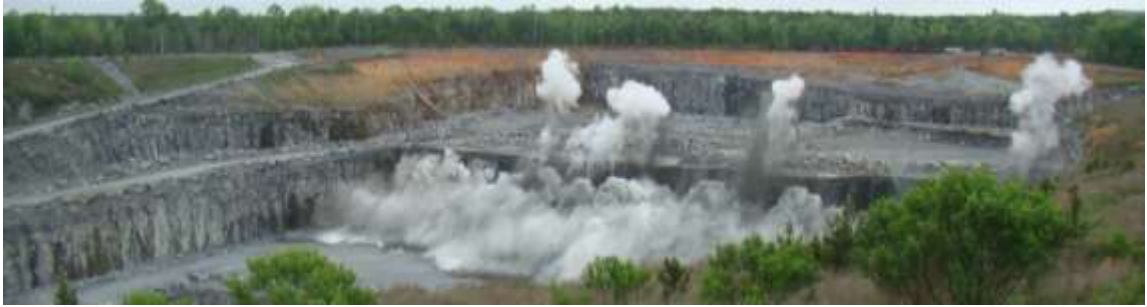
Figure E. 1: April 16, 2015, Shot 1 Blast Photographs
