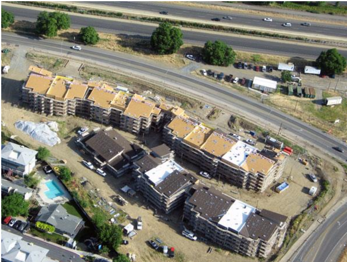
Figure 25: The New Harmony Affordable Housing Development in Davis. Source: http://www.mutualhousing.com
