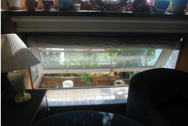
Figure 15: This "win-door" allows warm air from a greenhouse to heat this building's interior in the winter.
