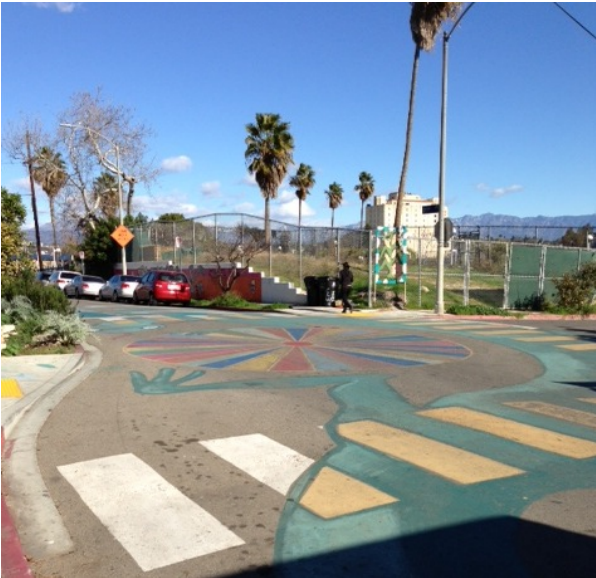
Figure 30: The intersection of Bimini and White House. Colorful pavement and bulb-outs enhance pedestrian safety.
