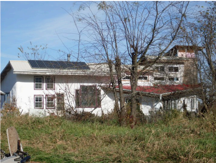
Figure 14: This larger timber-framed and straw bale dwelling (under construction in this image) is the home of a family with three children. Its interior footprint is smaller than a conventional home with the same exterior footprint, as straw bale insulation results in very thick walls.
