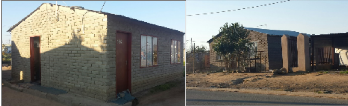
Figure 6: Houses from Botshabelo 900 Pamper Construction Project
