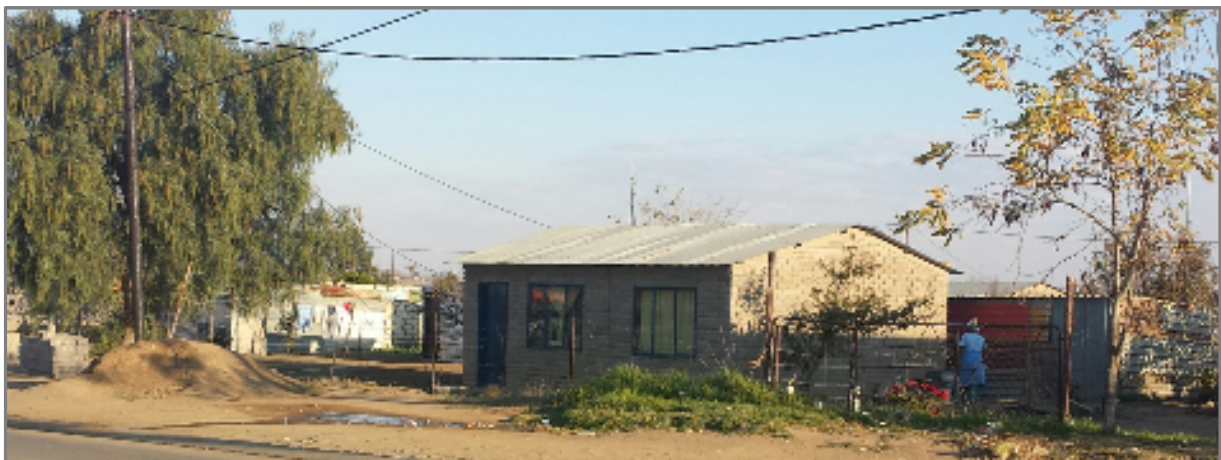
Figure 8: Botshabelo 900 Pamper Construction Project House
