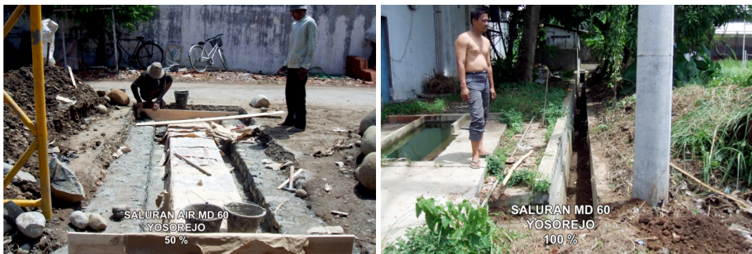
Picture 3. Local residents constructing the drain outlet outside factory wall
