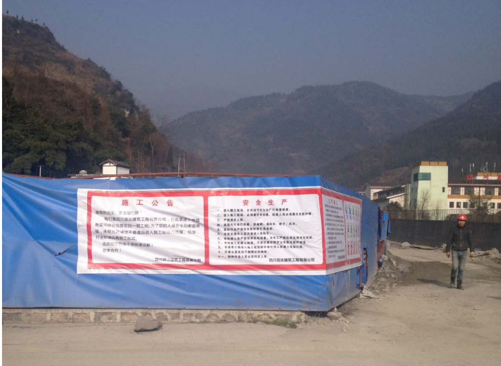
Figure 18 Construction Site of the Shouxi Lake Hazard Mitigation Project
