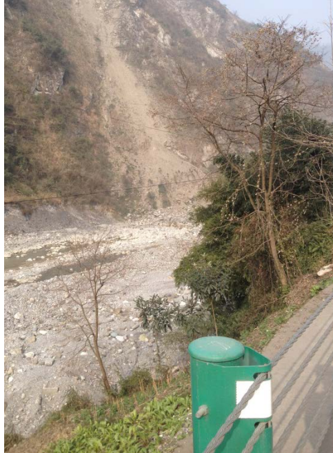
Figure 20 Pillars and Ropes on the Side of Highway to Prevent Pedestrians from Falling Down
