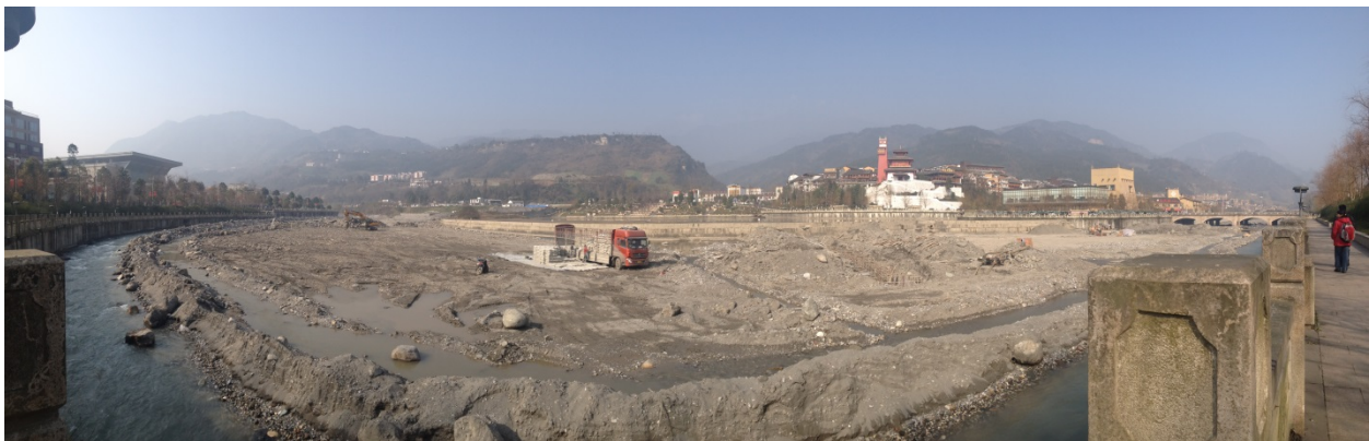
Figure 17 Shouxi Lake under Construction
