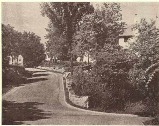
FIG. 9 RESIDENTIAL "CHARACTER" AS EXHIBITED IN THE "COUNTRY CLUB DISTRICT" NEAR KANSAS CITY, MO. Courtesy of the J. C. Nichols Companies
