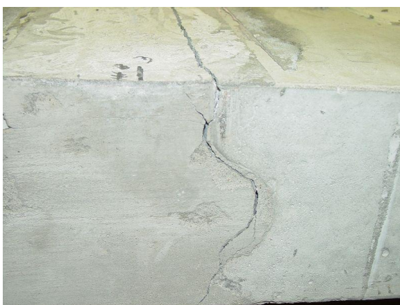
Cracking at closure region
