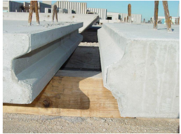
Shear key detail
