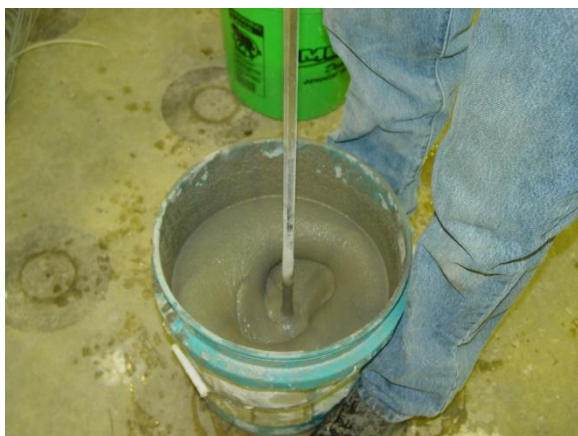
Mixing grout using power drill
