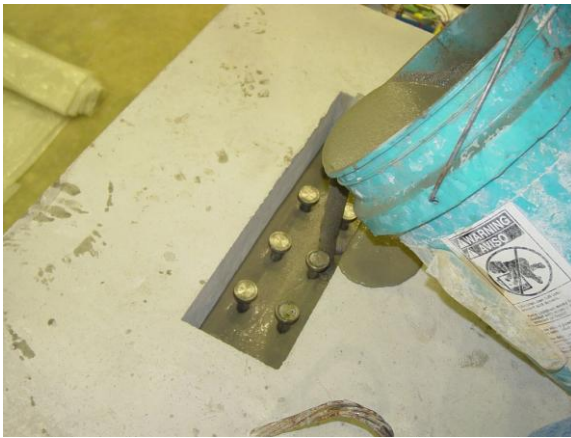
Grouting shear studs blockout
