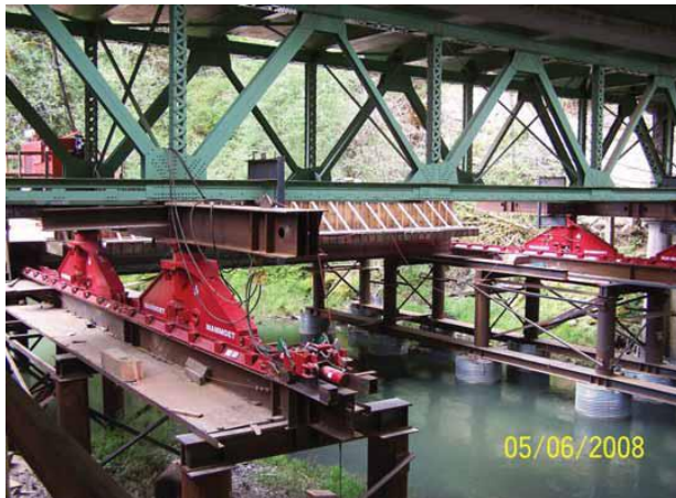
View of a complete hydraulic sliding system
