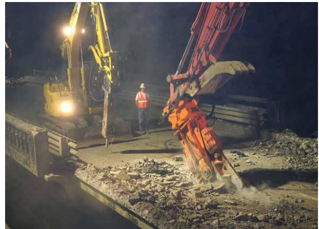
Demolition and dismantling of end panels
