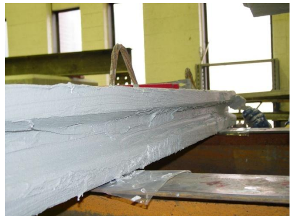
Epoxy matching cast shear key
