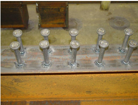
Shear studs
