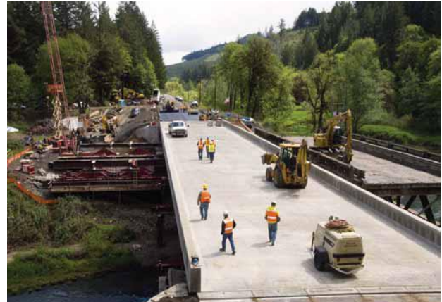
Replacement of superstructure and end panels.
