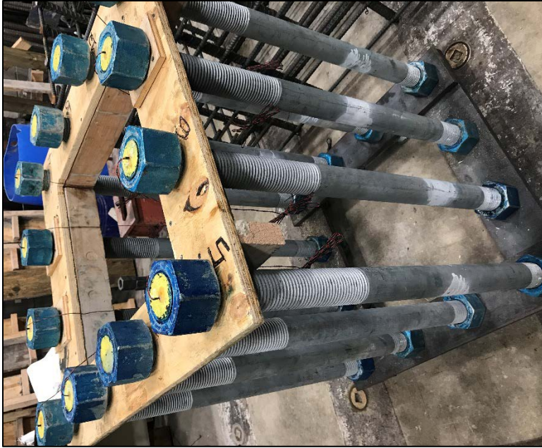
Figure 3.28 - Anchor Bolt Cage
