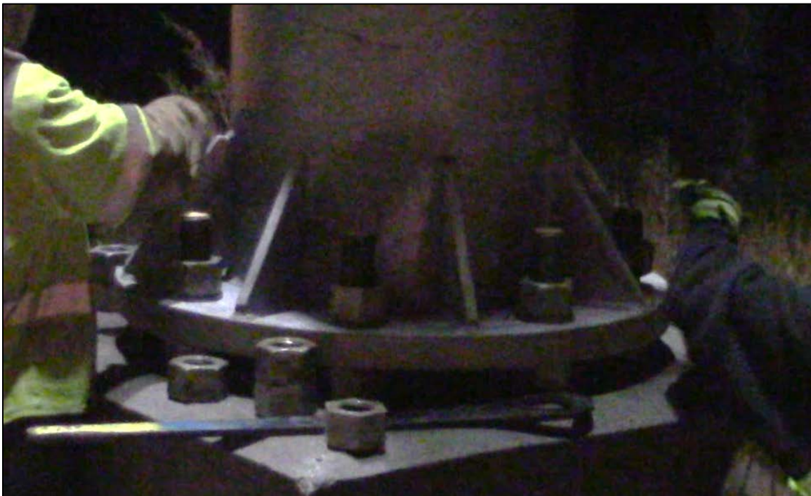
Figure 1.26 - Hand Tightening of Bolts
