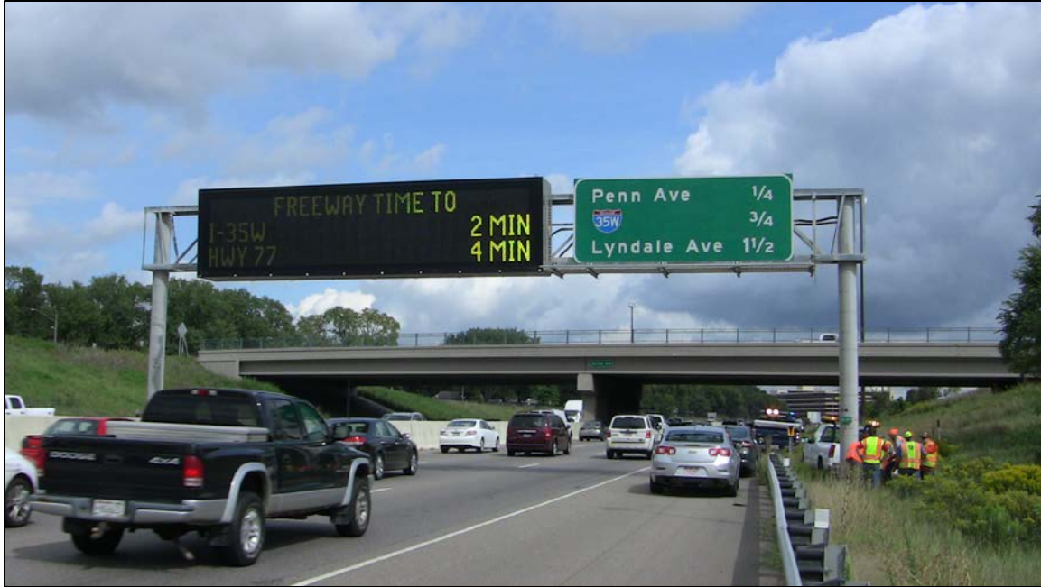
Figure 1.17 - VMS Support on I-494 Near I-35
