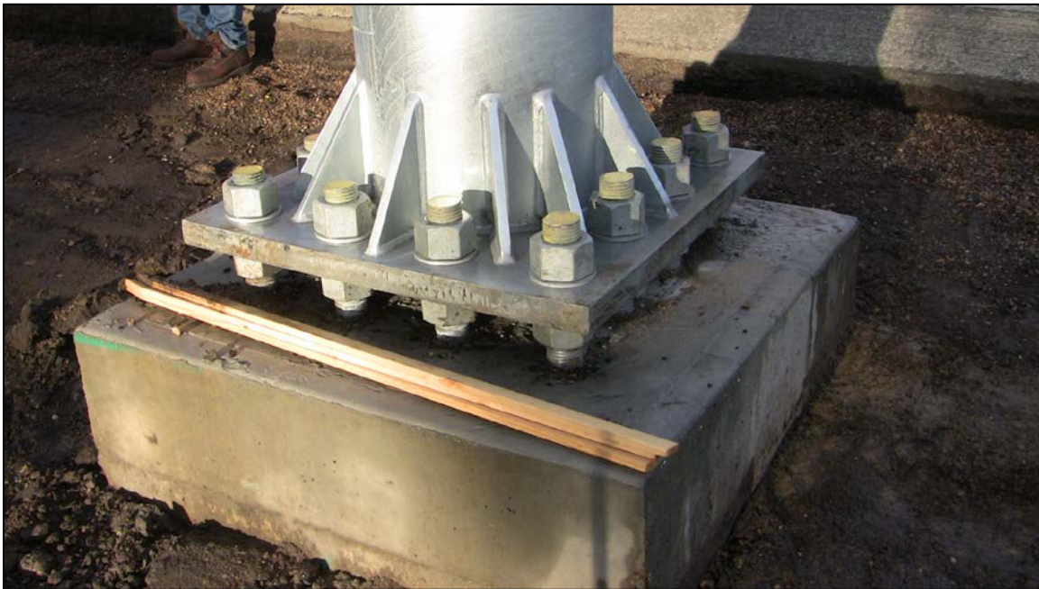
Figure 1.10 - Overhead Truss Baseplate and Anchor Bolts
