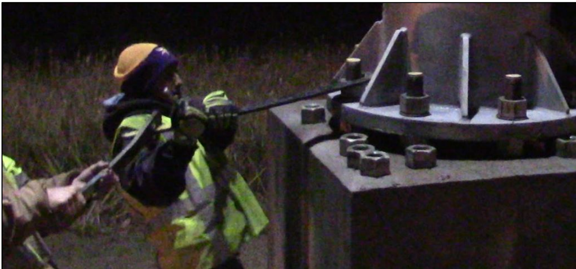
Figure 1.28 - Final Tightening After Making Reference Marks
