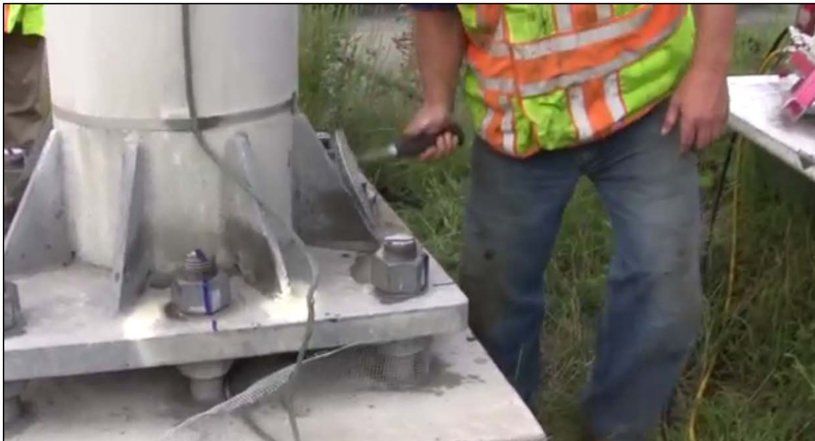
Figure 1.18 - Washers Struck to Inspect Nut Tightness
