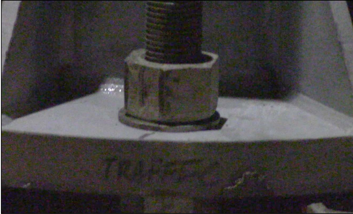
Figure 1.29 - Post Tightening with Reference Marks Shown
