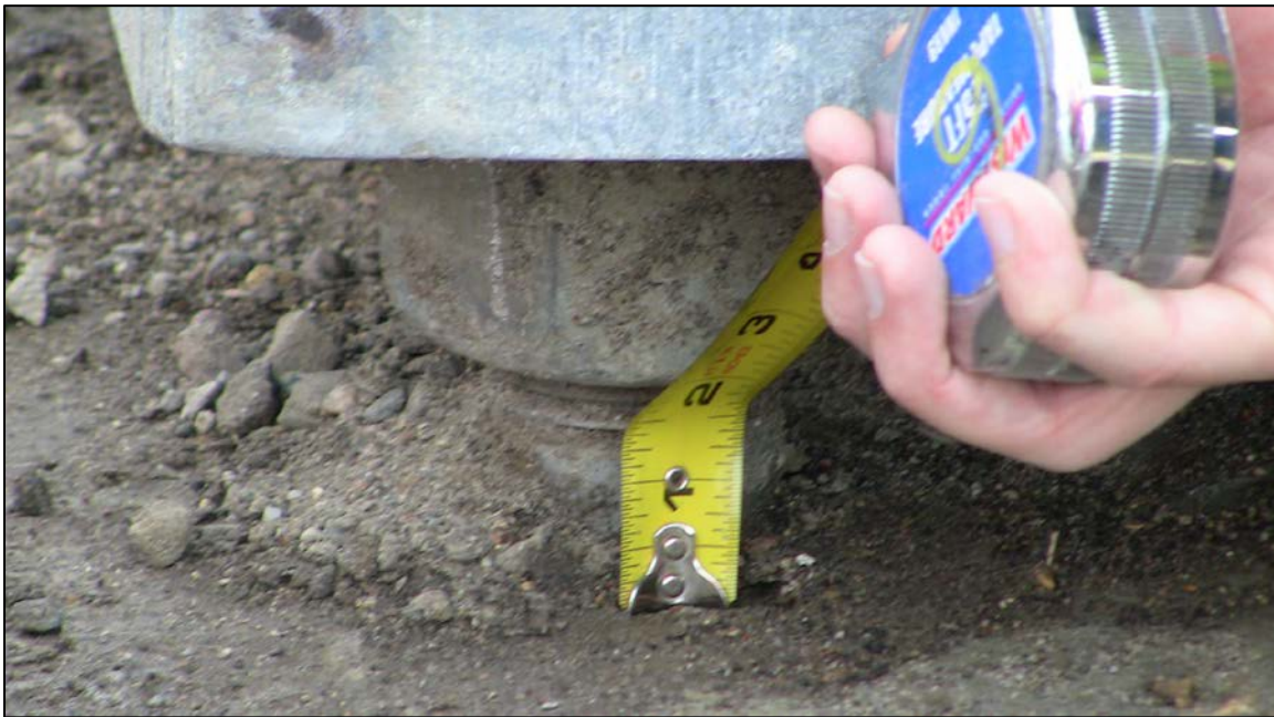
Figure 1.16 - Distance from Foundation to Bottom Leveling Nut
