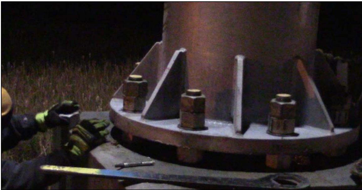
Figure 1.30 - Final Assembly with Jam Nuts
