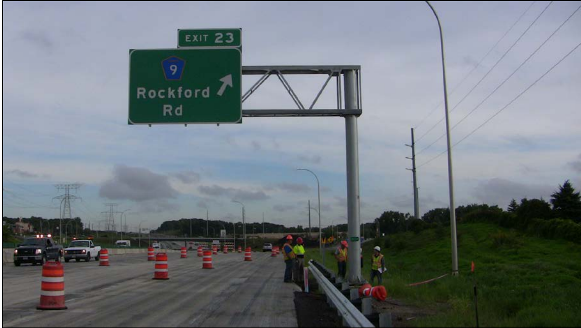
Figure 1.11 - Cantilevered Sign Support on Interstate 494 Near Maple Grove
