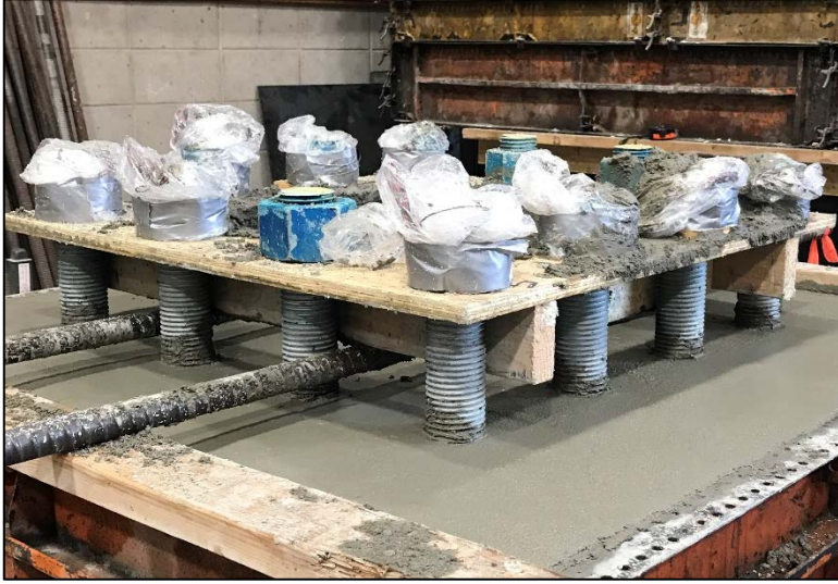
Figure 3.30 - Anchor Bolts during Concrete Curing
