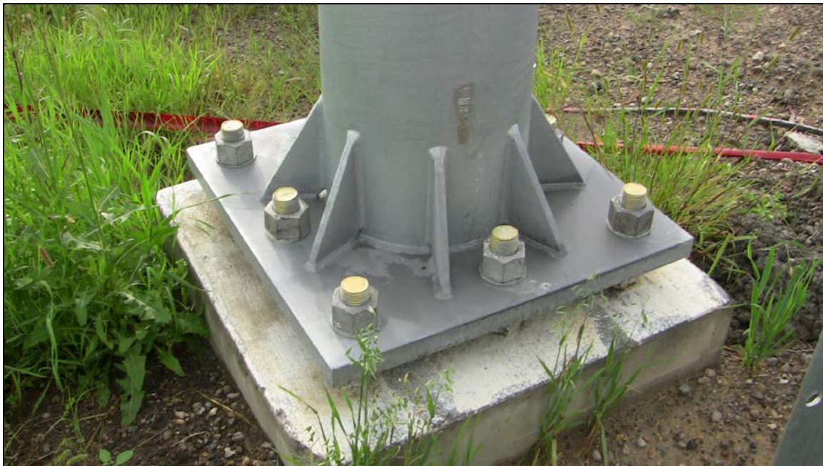
Figure 1.12 - Cantilevered Sign Support Baseplate and Anchor Bolts
