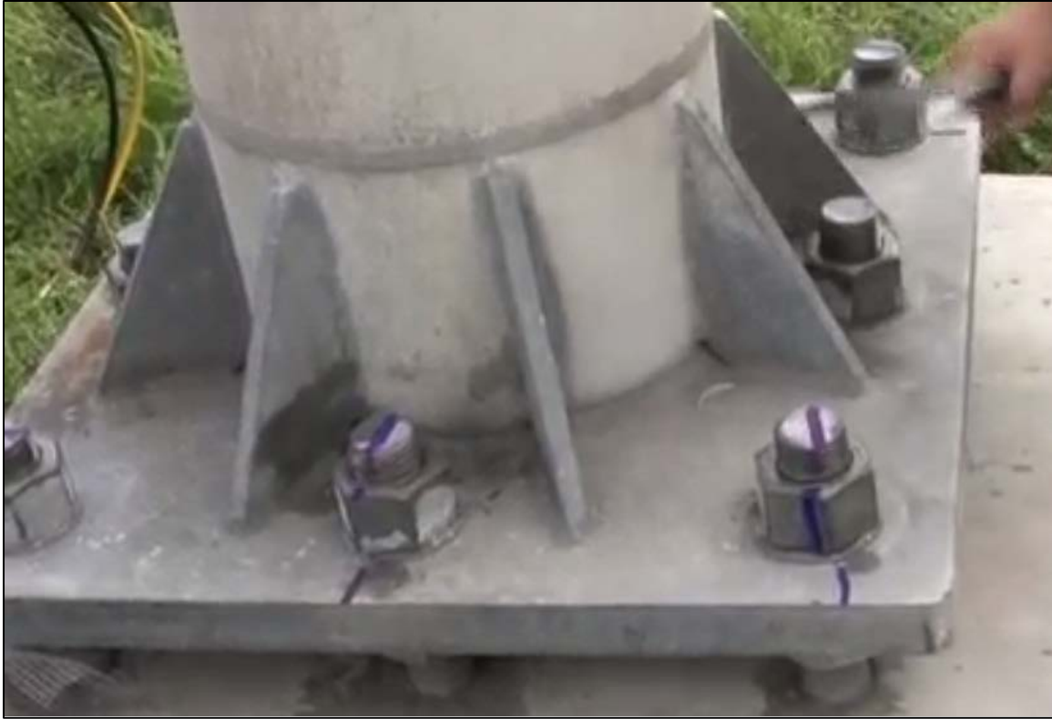
Figure 1.21 - After Maintenance Retightening
