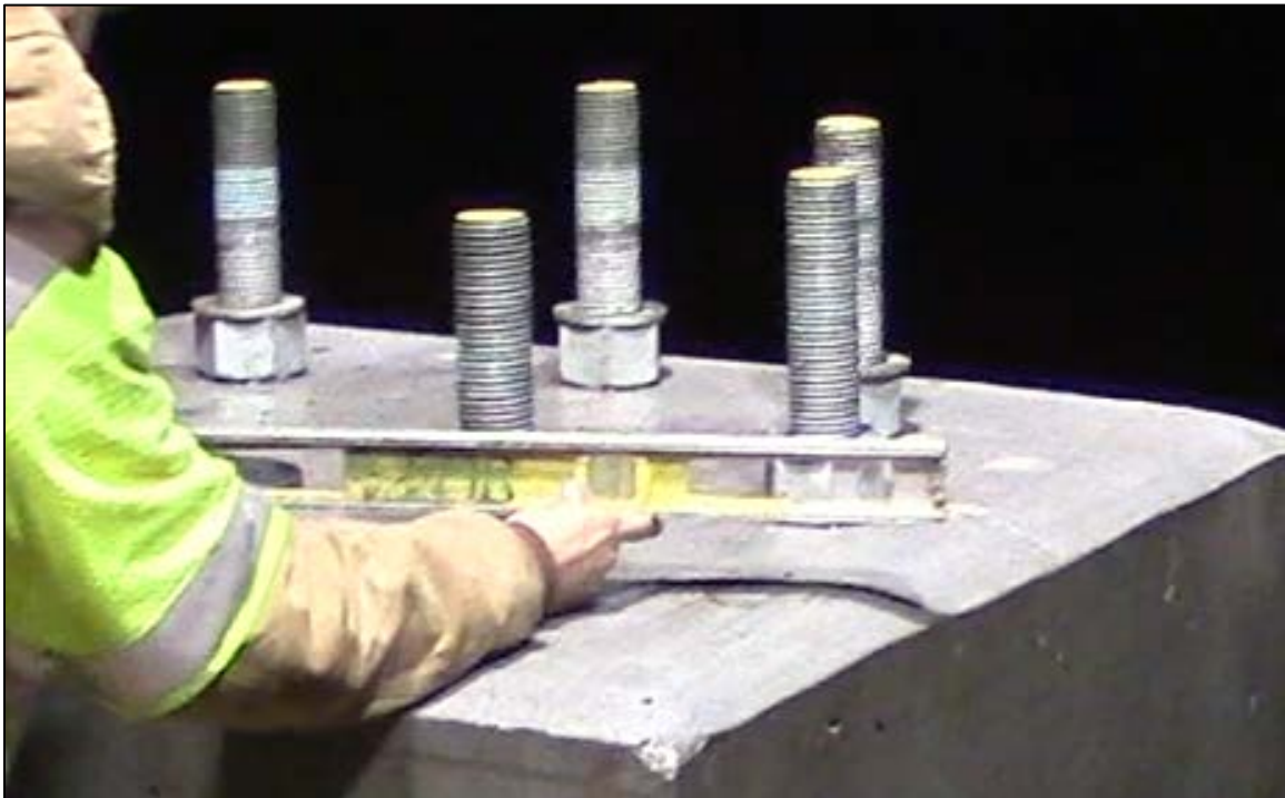
Figure 1.24 - Preparing for Pole Installation
