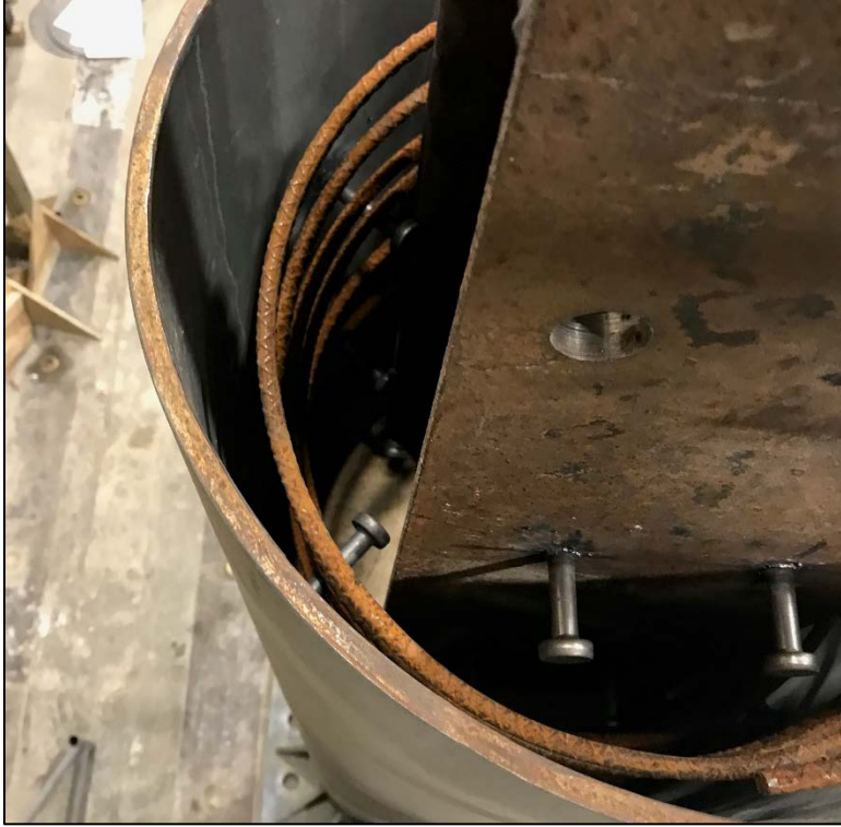
Figure 3.32 - HP10x57 and Confinement Placed in Sign Post
