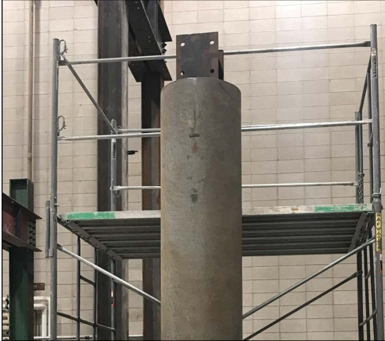
Figure 3.33 - H-Pile Placed Inside Sign Post
