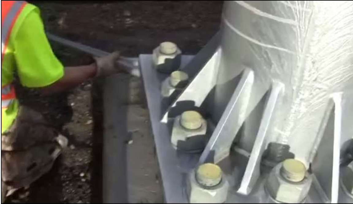
Figure 1.13 - Leveling Nut Tightening in Minnesota
