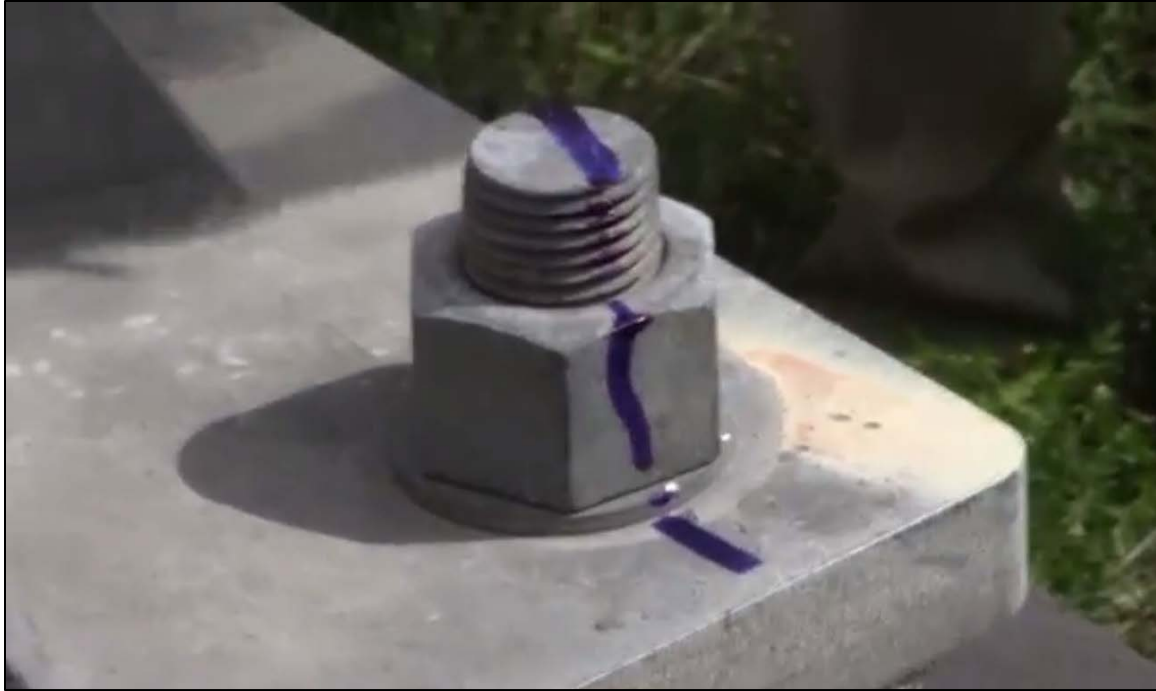
Figure 1.19 - Reference Marks Used During Maintenance
