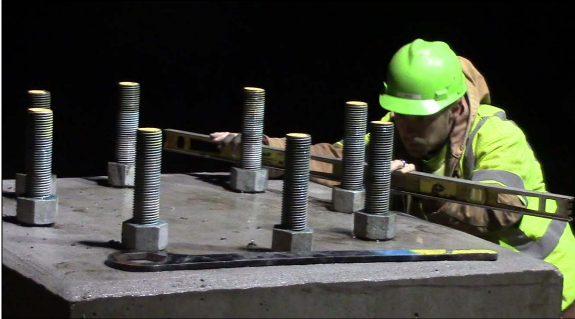
Figure 1.23 - Leveling During Iowa Site Visit
