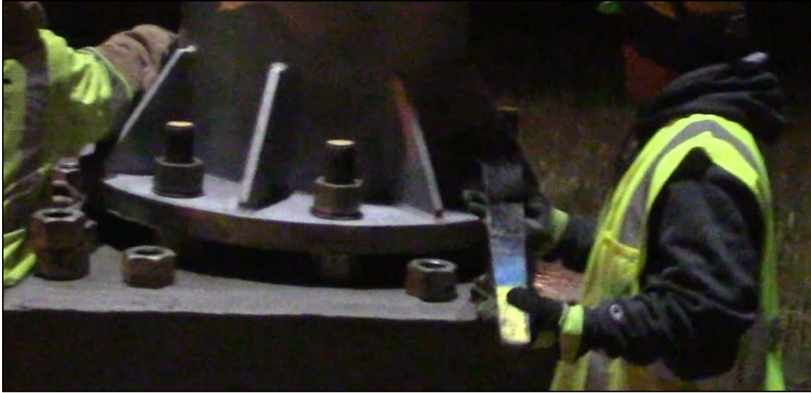
Figure 1.27 – Snug-tightening of Bolts
