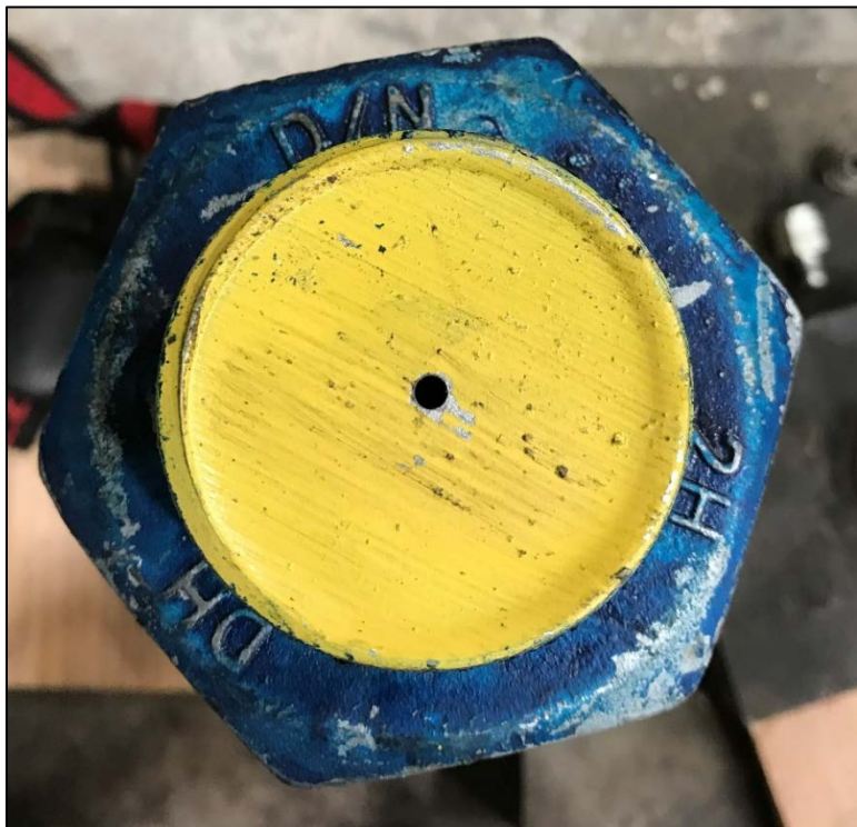
Figure 3.5 - Predrilled Hole in 2-1/4" Anchors
