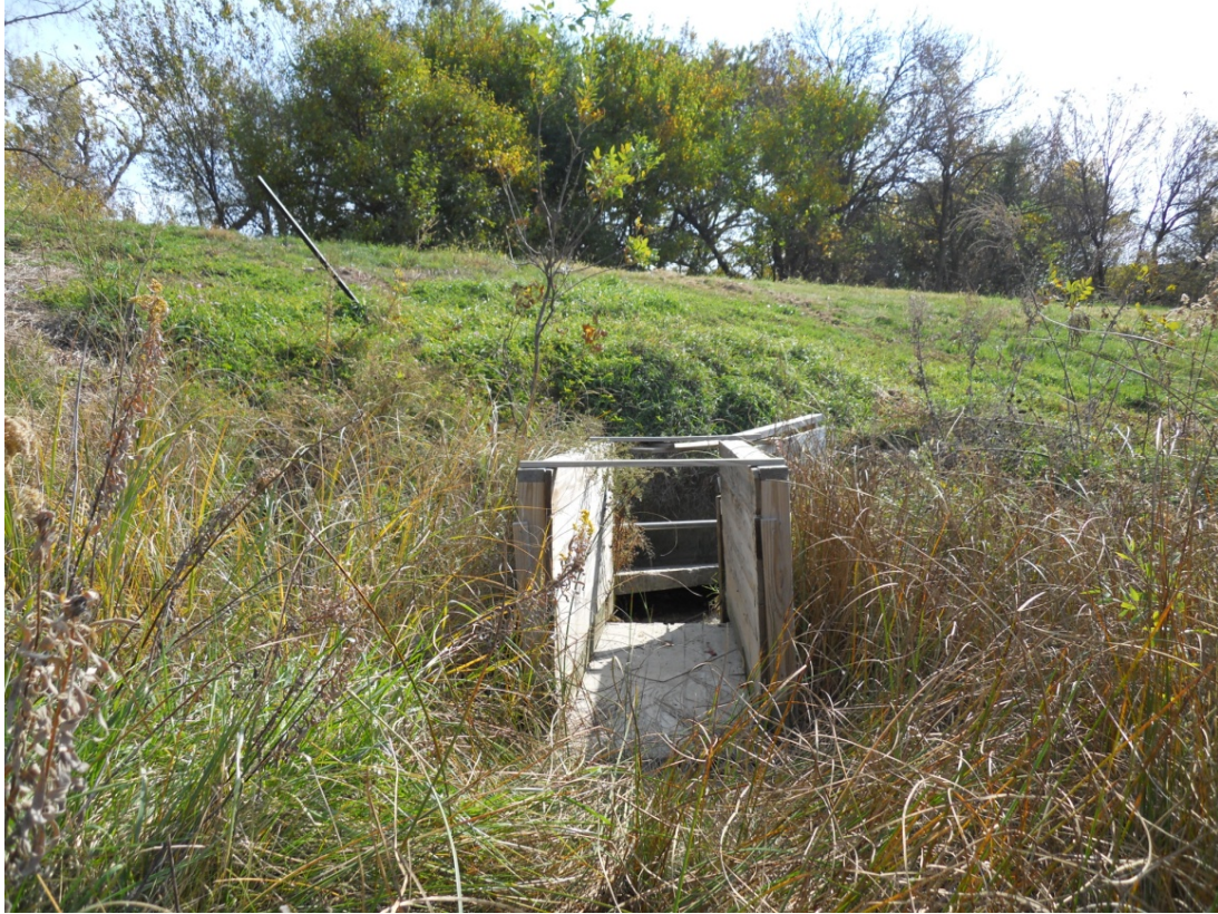
Figure 4-5: Rectangular Flume Installed at Site E
