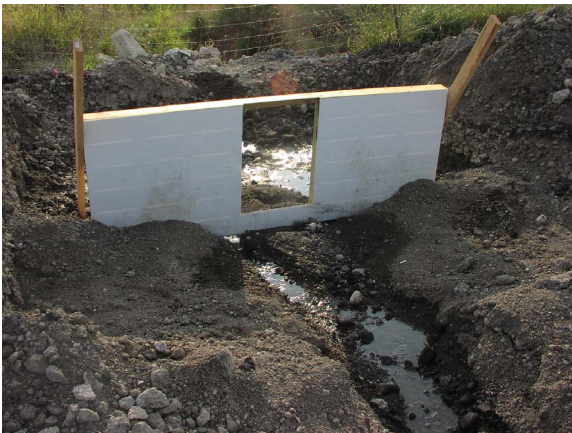
Figure 4-3: Rectangular Weir Installed at Site A
