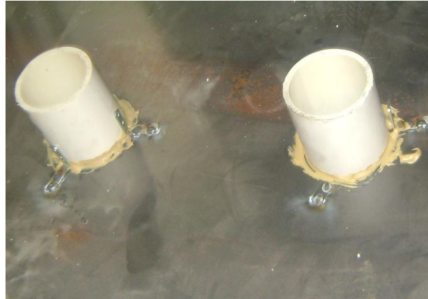
Figure 52: PVC Grout Holes
