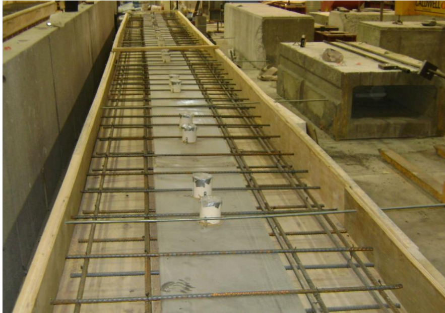
Figure 54: Formwork and Deck Reinforcement for DCA Specimen
