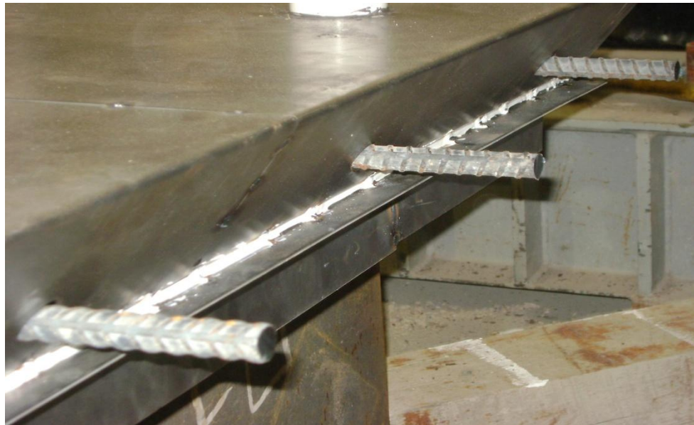
Figure 25: Deck Reinforcement
