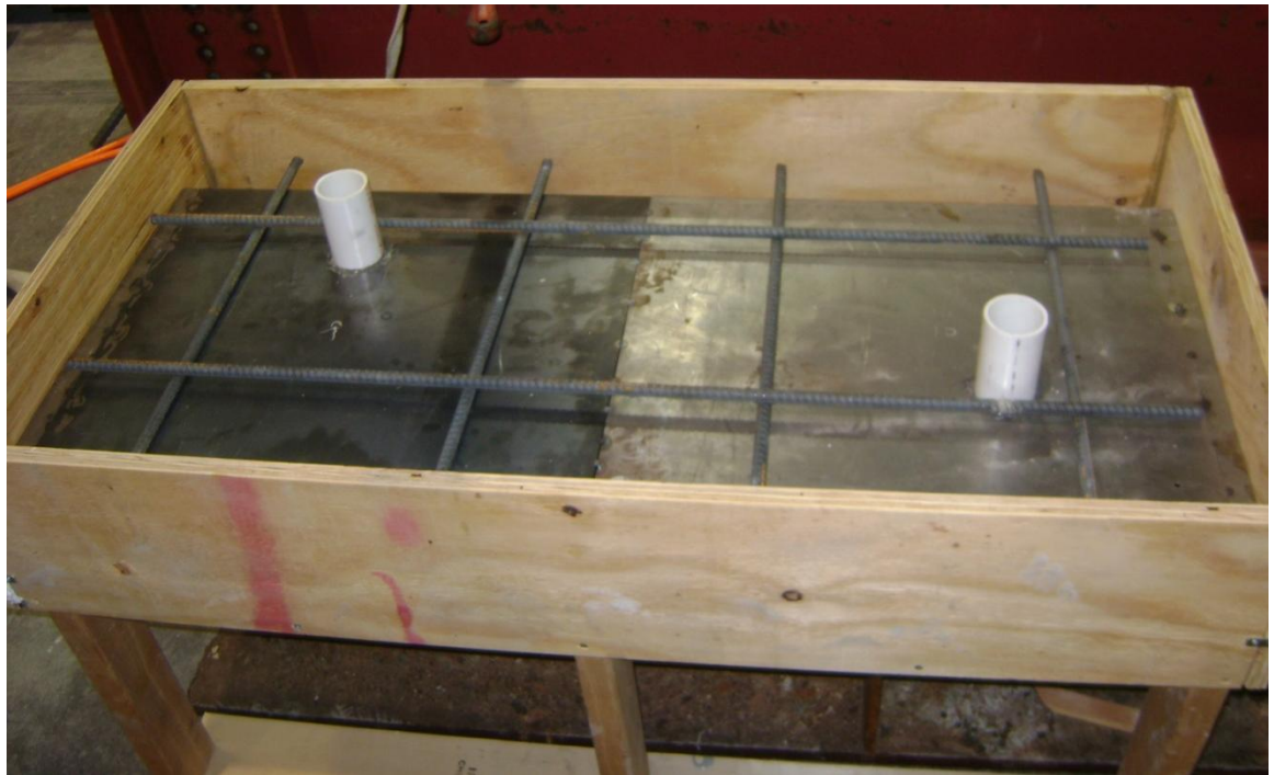
Figure 26: Complete System before Pouring
