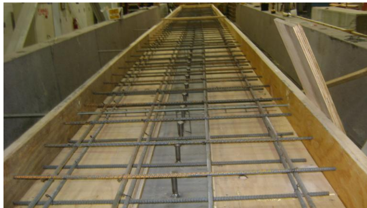
Figure 53: Formwork and Deck Reinforcement for Specimen without DCA
