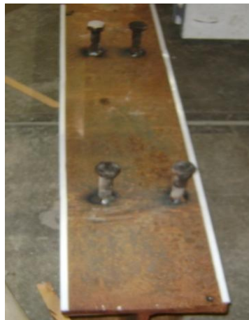
Figure 21: Girder with HDPE Strips
