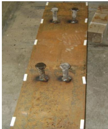
Figure 20: Girder with Teflon Strips
