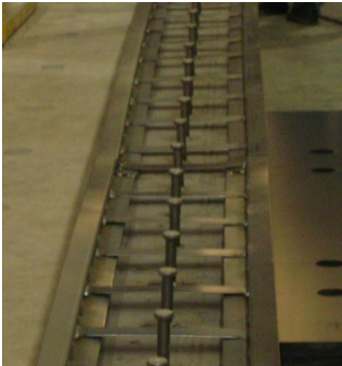
Figure 49: Welded Support Angles
