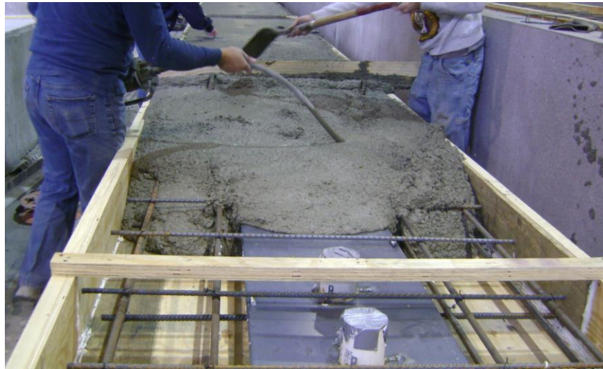
Figure 55: Pouring of DCA Specimen
