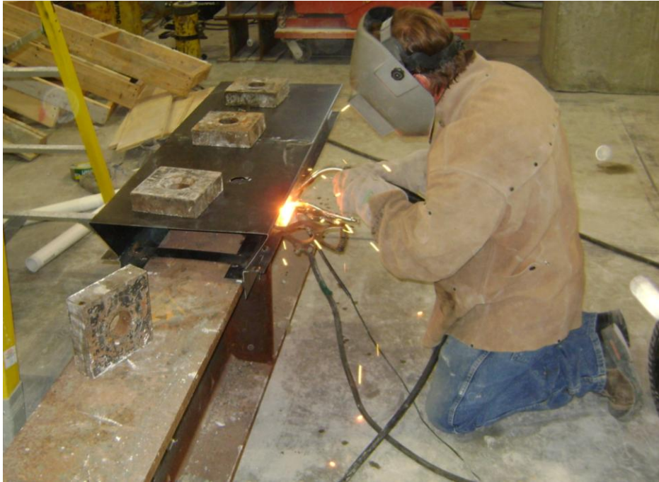
Figure 32: Welding of Specimen
