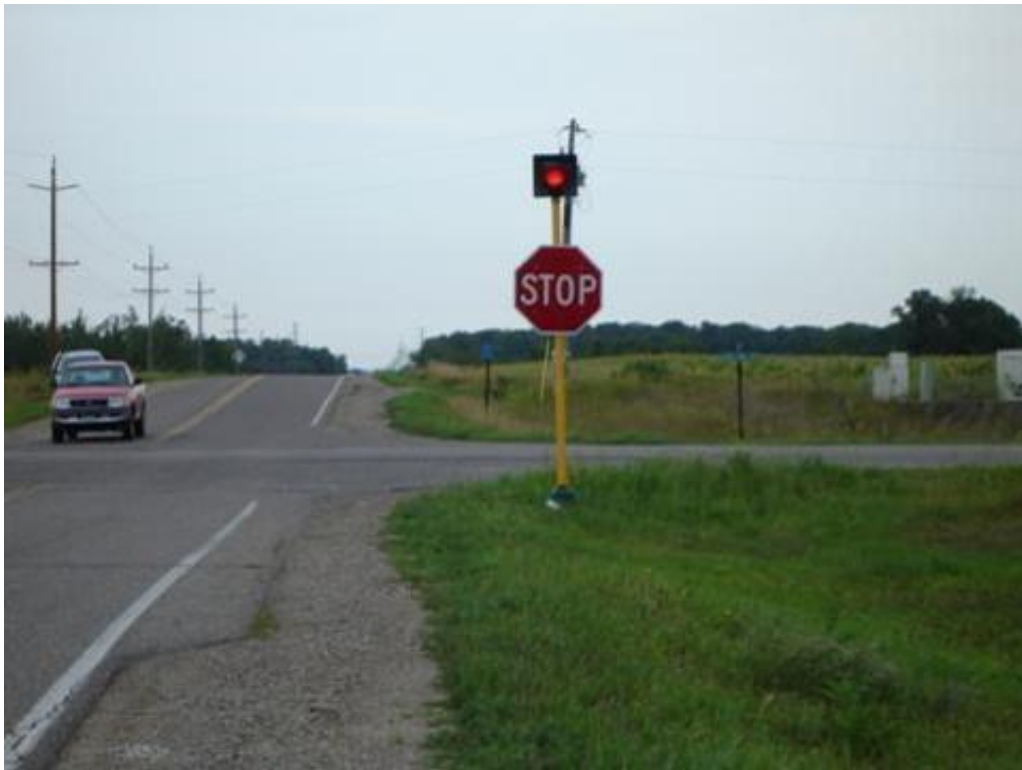
Figure 3-11: Flashing beacons at rural intersection source: Stein and Neuman 2007
