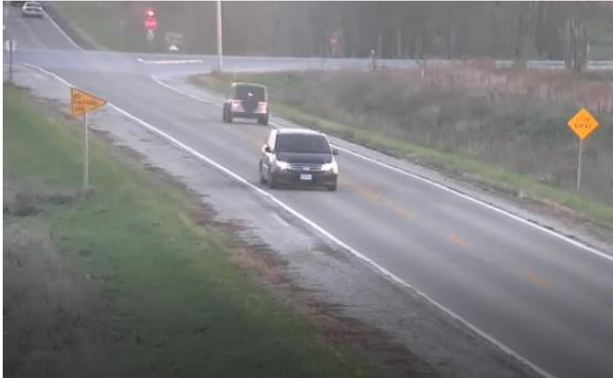
Figure 4-8: Beacon shown as active as the subject car approaches the intersection in Dallas County
