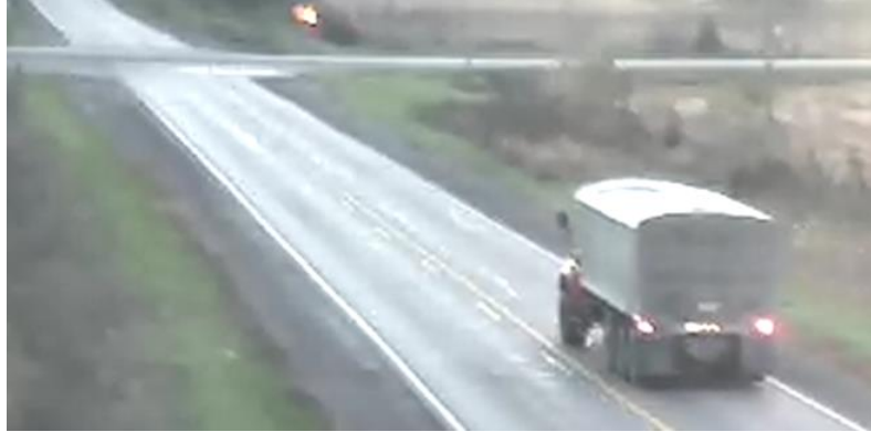
Figure 3-7: Beacon illuminated at the south approach of Hwy 1 and 140th Street.
