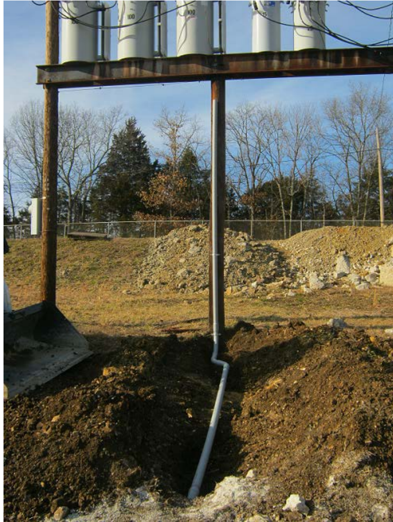
Figure 7.15. Surface preparation to pass the power cable underground
