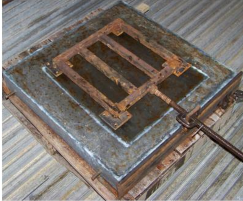
Figure 3.10: Applying Acrylic Sealant on Concrete Slab
