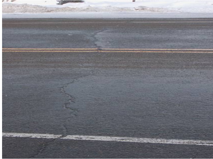
Figure 2.20 - Thermal cracking
