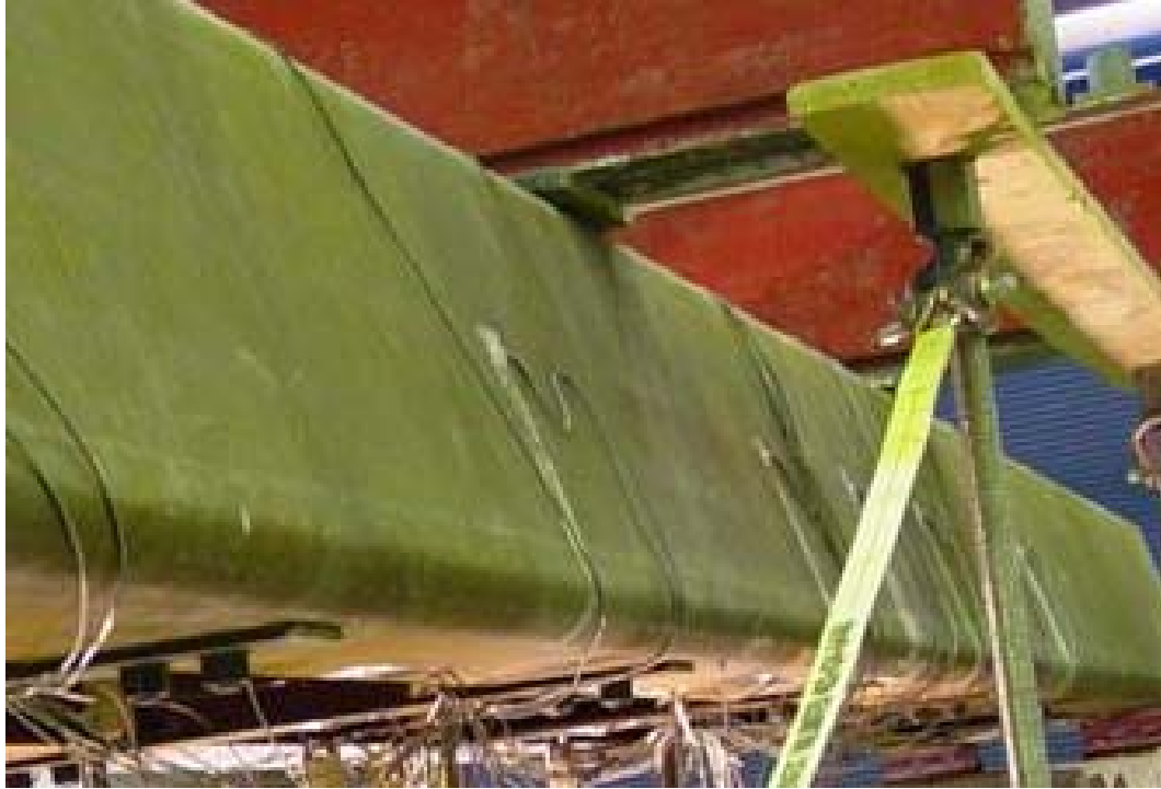
Figure 3-8 Girder web before loading
