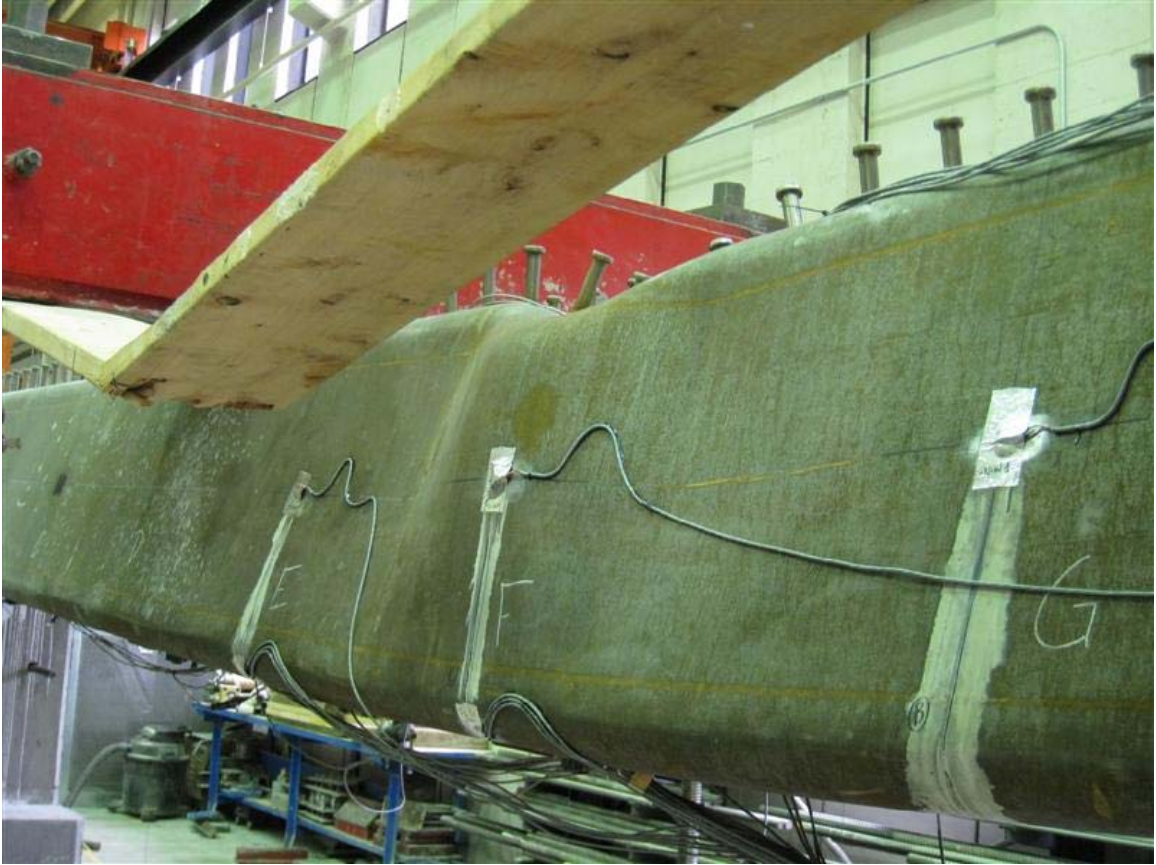
Figure 3-49 Girder permanent deformation after unloading. Web buckling
