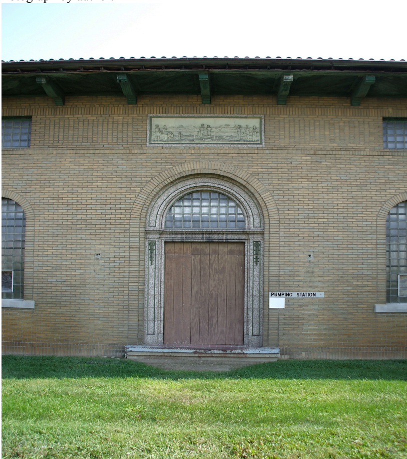
Figure 10. Pump House front view, Belmont Advanced Wastewater Treatment Plant, 19 September 2007. Photograph by author.
