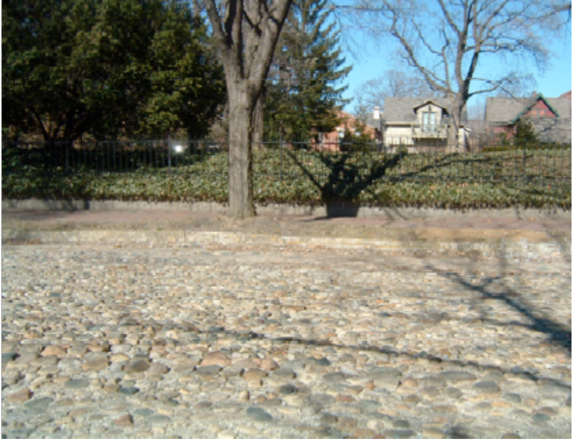
Figure 2. Cobblestone surface in the 500 block of Lockerbie Street, Indianapolis, Indiana, February, 2006. Photograph by author.
