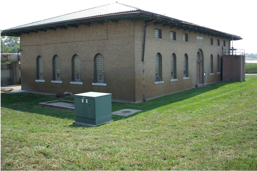
Figure 9. Pump House exterior, Belmont Advanced Wastewater Treatment Plant, 19 September 2007. Photograph by author.
