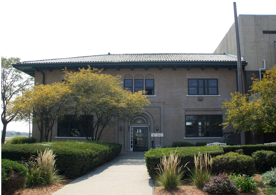
Figure 11. Administration Building, Belmont Advanced Wastewater Treatment Plant, 19 September 2007. Photograph by author.
