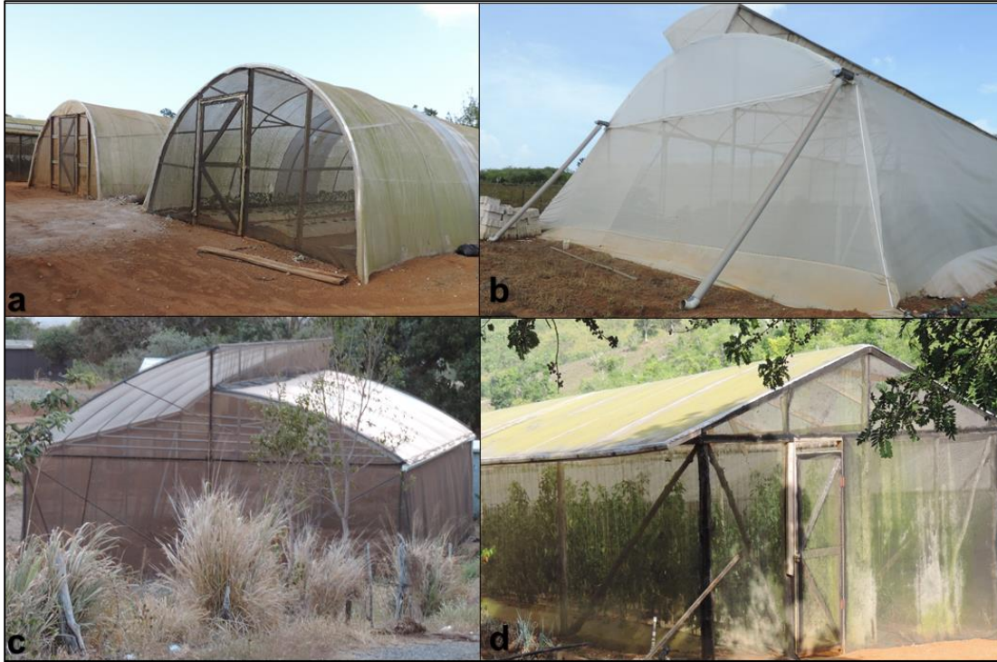
Figure 4.4. Greenhouse Designs: a. hoop-house; b. double-ridge house; c. Single ridge house; and d. gabled house
