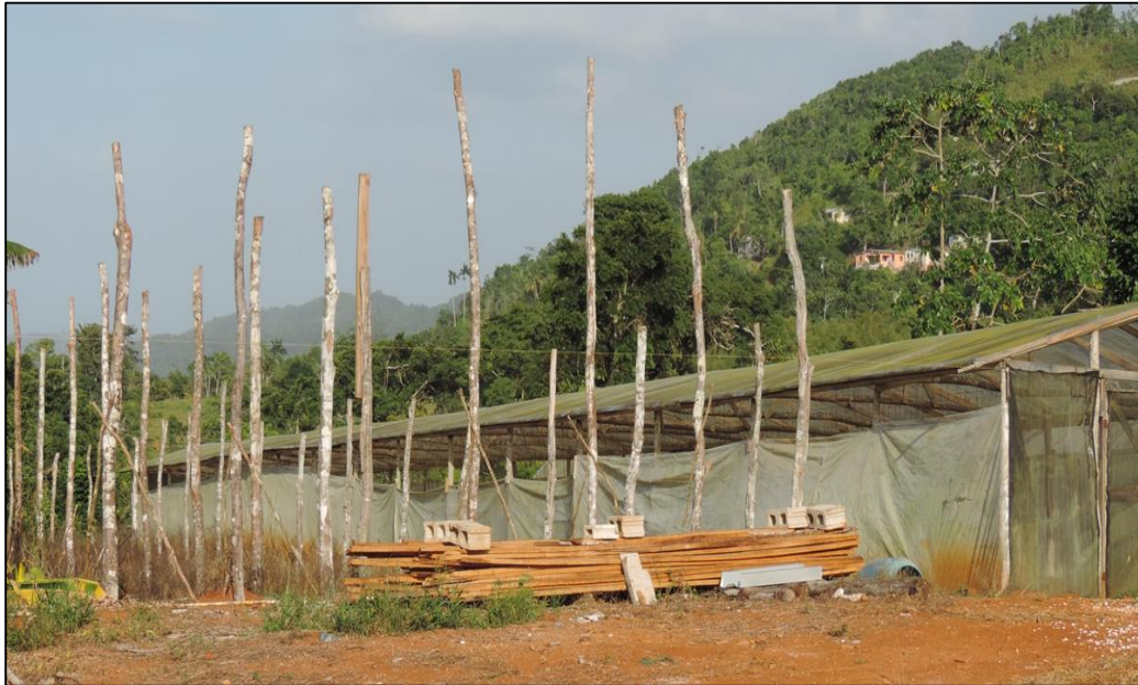
Figure 4.3 Wooden greenhouse under construction, St. Ann
