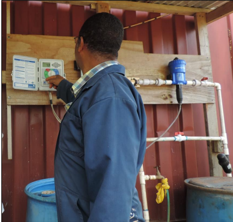
Figure 7.1 Greenhouse farmer demonstrating the use of his automated fertigation system
