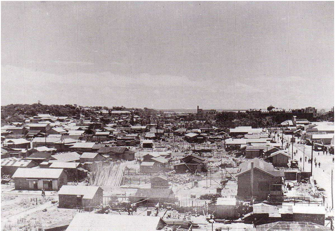
Fig 6.2: Azuma-chō August 1946. About half of the razed plots now have new structures. This part of the city had been largely rebuilt a second time by the early 1960's.
