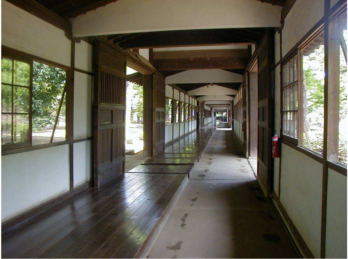
Fig. 4.8: Internal and external use combined. The raised highly polished wooden floor is for monks wearing slippers, the concrete for visitors in outdoor shoes. Sōjiji Temple, Tsurumi [IR]
