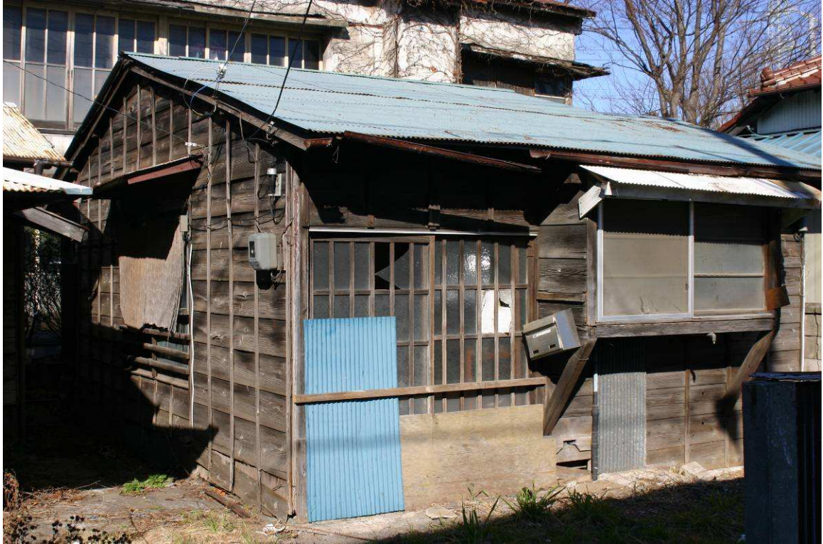
Fig. 6.8: Carpenter constructed house from about 1952. Before tin cladding was available for plywood cedar shingles continued to be used for exterior cladding. Shioda-chō
