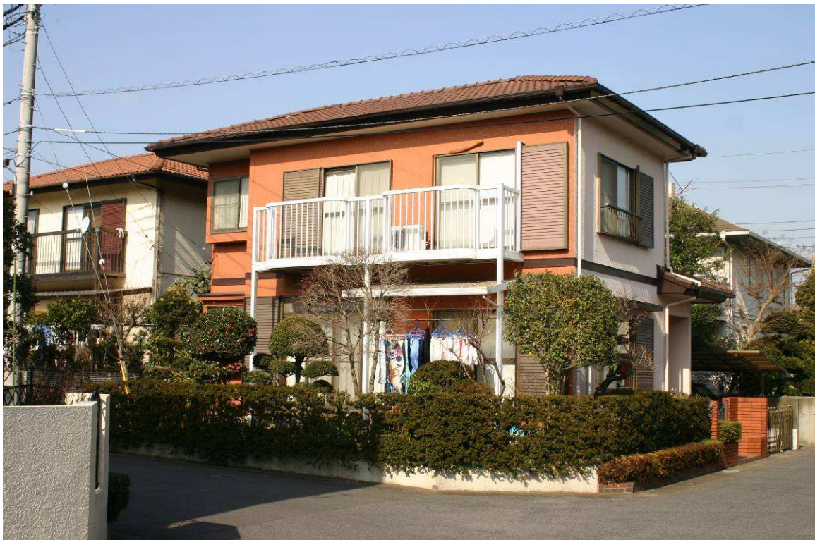
Fig. 8.9: Typical two storey owner occupied home from about 1980. Wooden structure with plywood skin protected by paint, standard components, and a car port. Higashi Chishirodai
