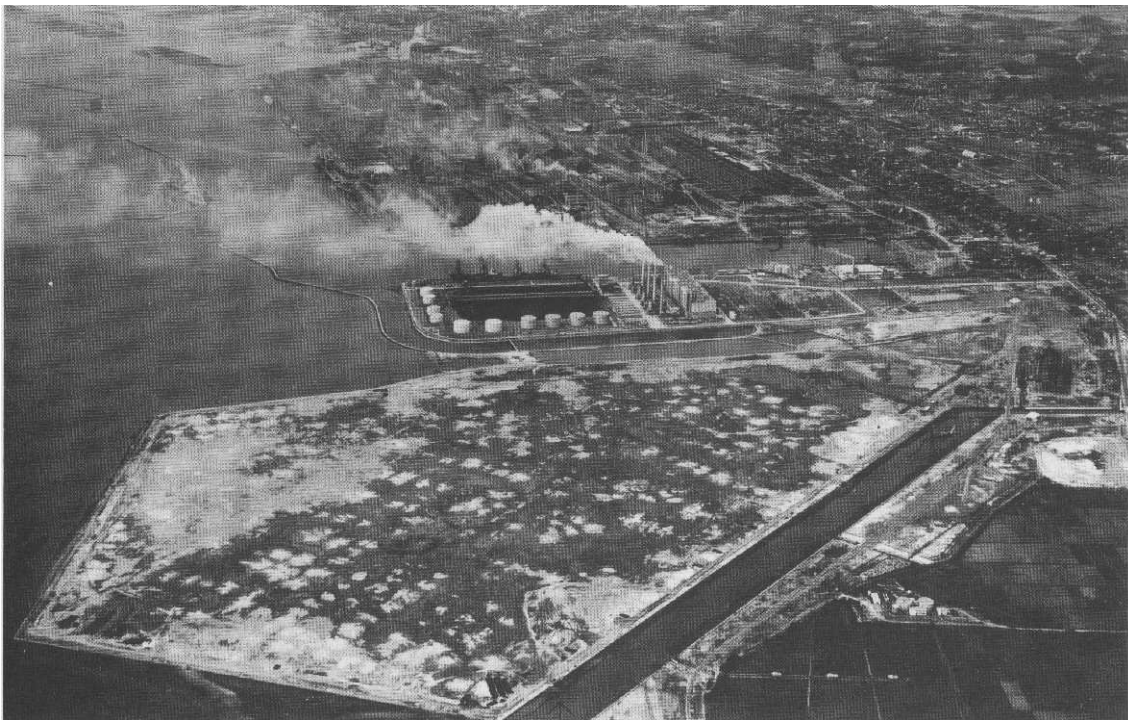
Fig 7.8. Classic 'kombinato'. 'Dredge reclamation' of additional new land for Kawasaki Steel at Niihama in 1963. The air pollution from the TEPCO coal power station and the Kawasaki Steel integrated site behind are obvious. The site is for new steel finishing processes.
