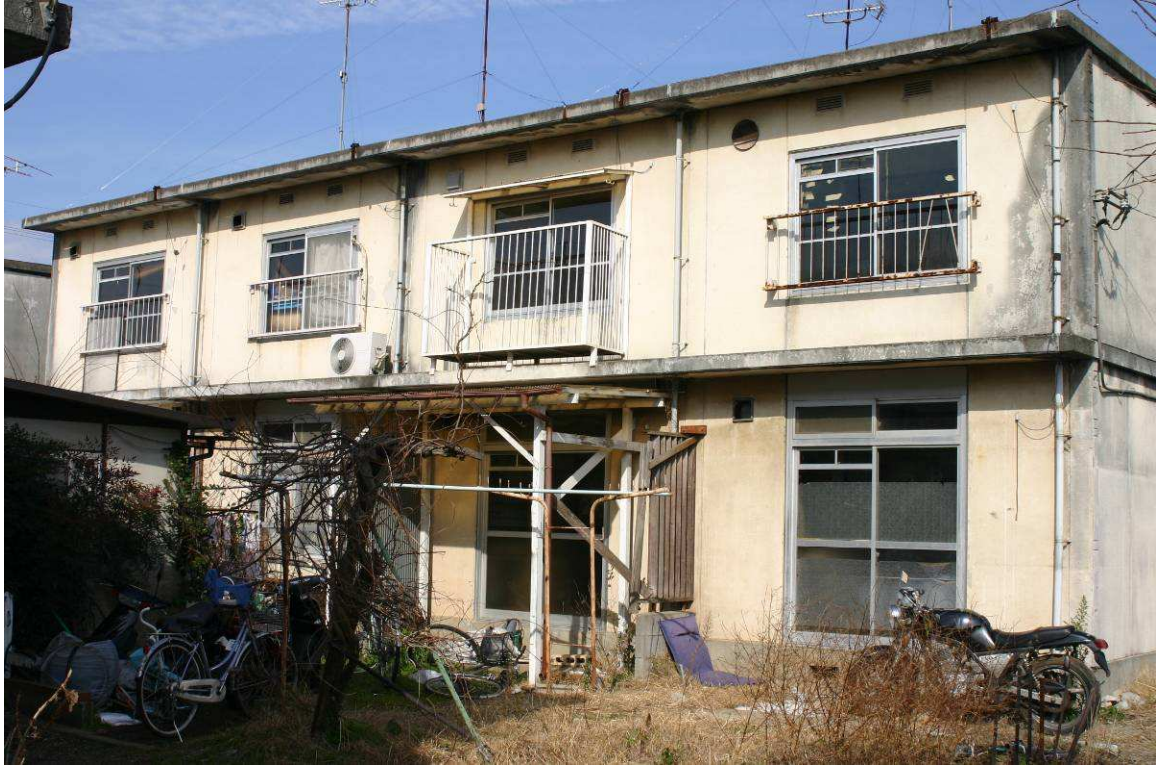
Fig. 6.9: Early wooden framed public housing. These survivors are 1960's nagaya (terrace houses). Earlier cheap apartments for steelworkers were similar structures. Chishirodai
