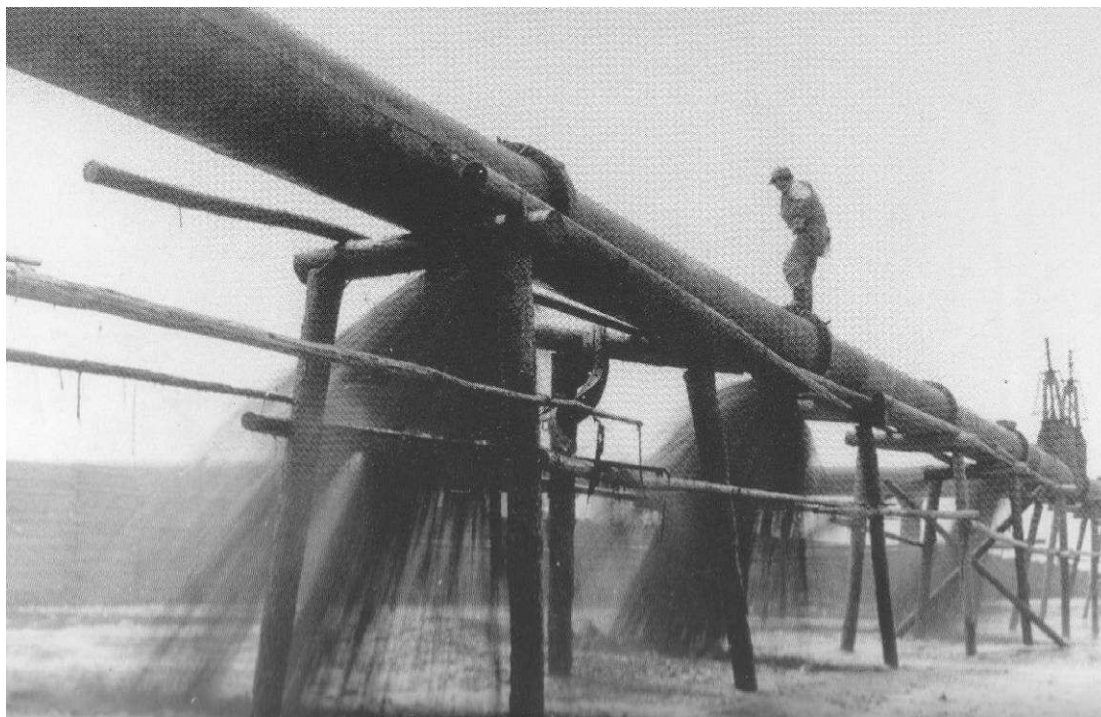
Fig. 7.2 'Dredge Reclamation' in progress on the foreshore at Inage 1964. This was the commonest technique used for landfill and consists of pumping silt dredged offshore into banded areas as slurry and allowing the material to dry out and solidify into new ground.
