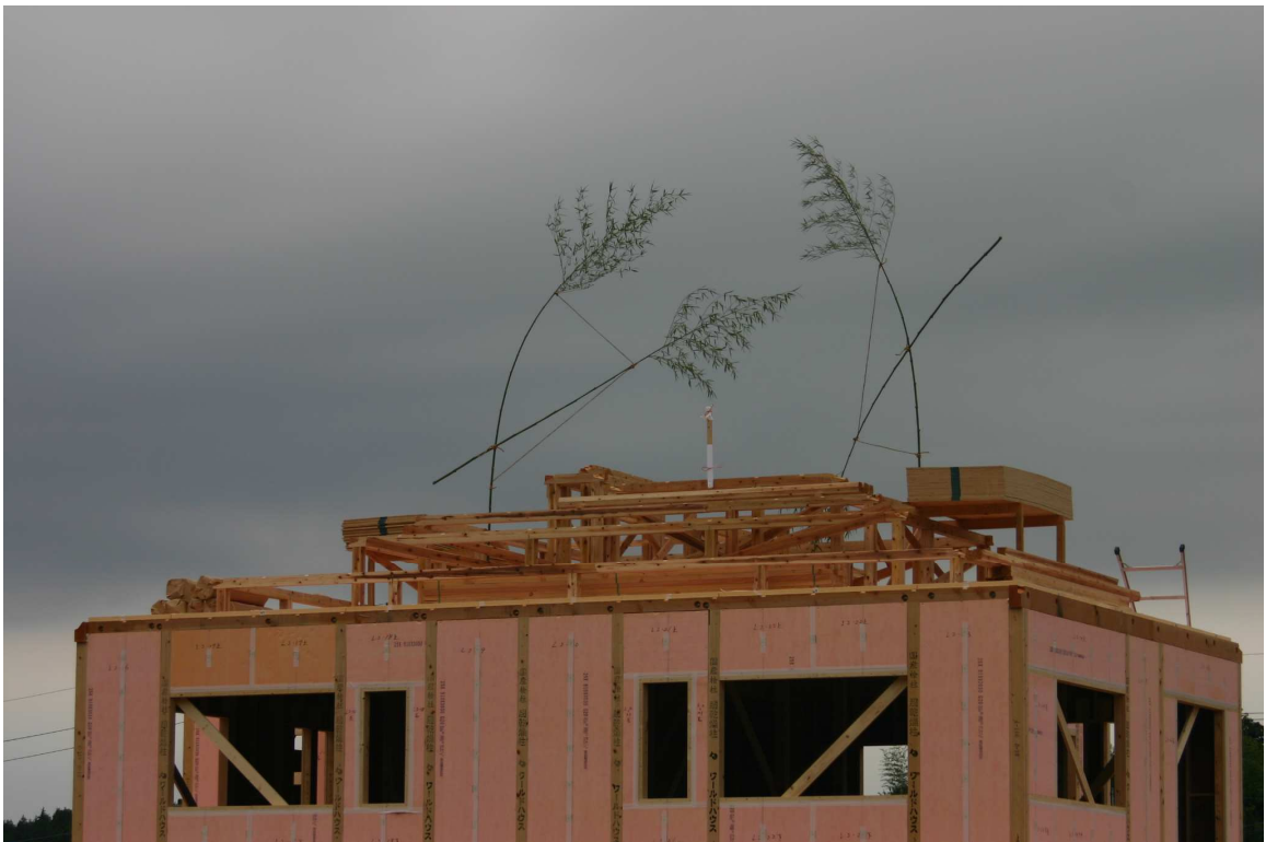
Fig. 4.4: House under construction decorated for a muneage-shiki ceremony. Sanmu-shi [IR]
