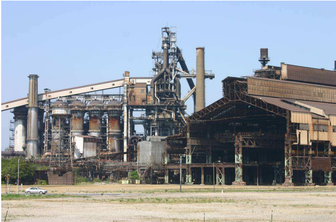
Fig.9.1: A changing order. In 2005 the first blast furnace and strip mill built in 1953 by Nishiyama Yataro are demolished in favour of a retail mall and a business innovation park.
