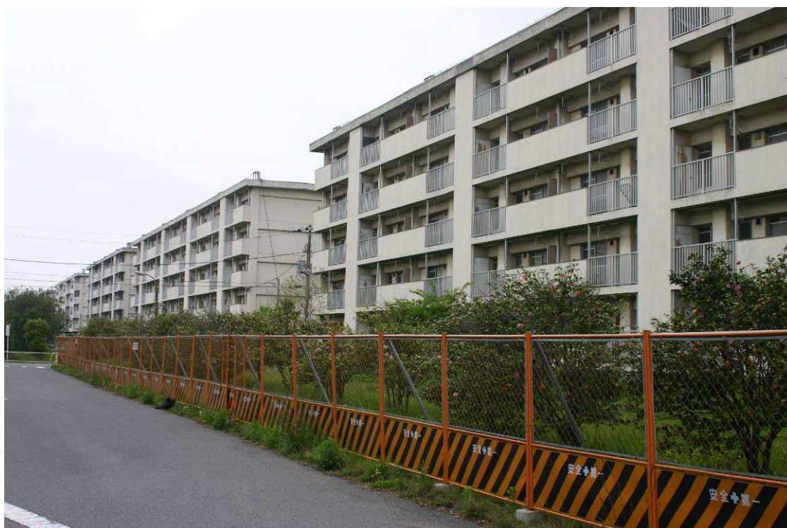
Fig 9.6: Some of the 730 late 1960's JHC apartment blocks vacated and sealed off ready for demolition and replacement by condominium clusters. Inage-kaigan 5-chome 2005. [IR]
