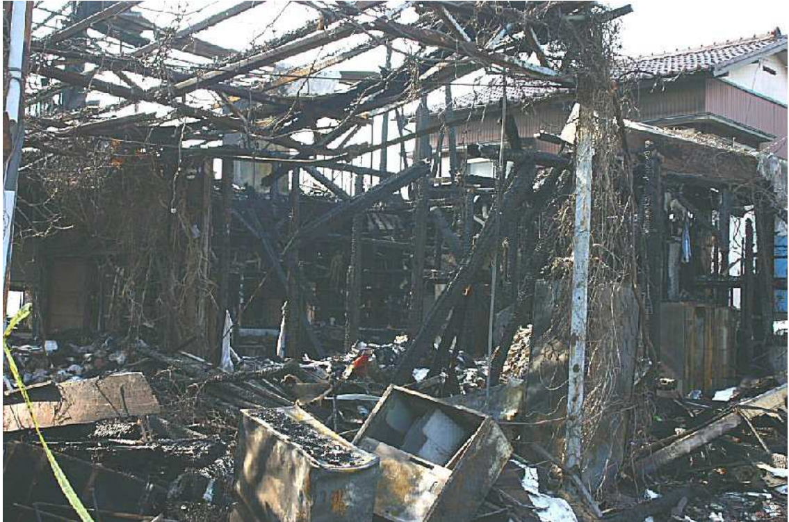
Fig.1.1. Even modern wooden framed dwellings are completely destroyed by fire within about twenty minutes. House fire at Nishi-Tsuga 4-chome January 2007
