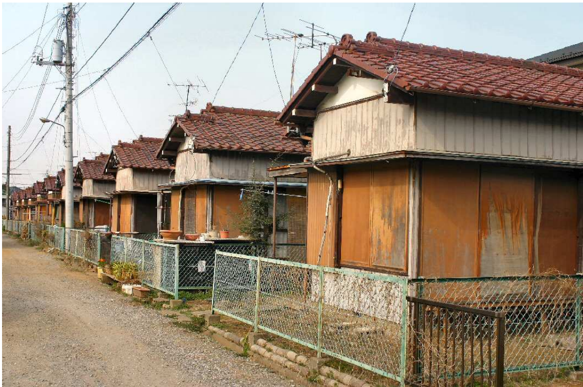
Fig. 7.11. Detached public dwellings built 1962, Miyanogi-cho. Until ferroconcrete construction became established JHUDC practice these 'late austerity' designs were still widely produced.
