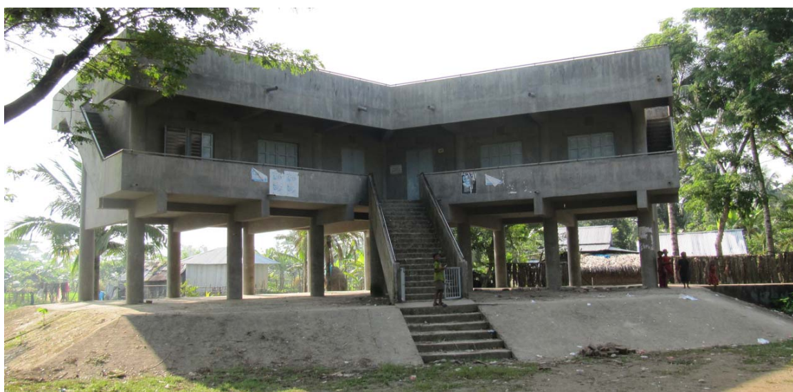
Figure 4.4: Gabtola Cyclone Shelter
