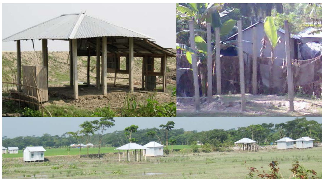
Figure 5.6: Abundance of abandoned houses – the construction cost (excluding material costs) for every single house was Taka 10,000, which make no sense now. All of the houses in a row in the bottom picture are now abandoned. (Source: Author)
