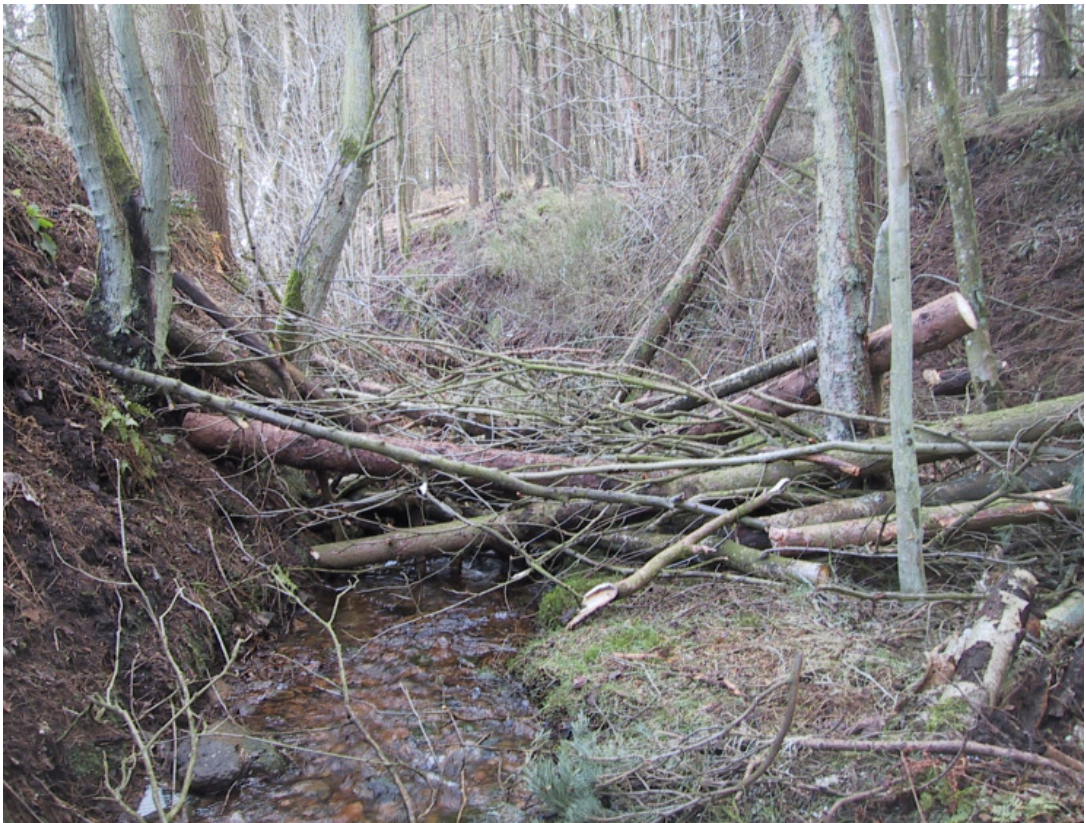
Figure 5.1 An artificially constructed large woody debris dam, in a river channel at low flow, Cropton, north of Sinnington, 25 th March 2010. The logs and branches that make up the dam have been wedged against trees to reduce the chance of being washed downstream in a flood. Vertical stakes can also be driven into the river bed in front of the dam for the same purpose (Forestry Commission, 2010). Photograph by Dr. Nick Odoni, Durham University.
