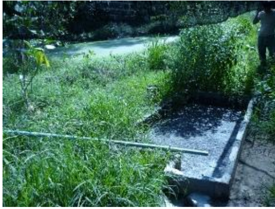
Photo 3. Pig waste pit and retention pond. After the removal of solids from the piggery floor, wastewater from flushing the pens is collected in a pit and a retention pond (left upper corner) with both showing signs of eutrophication. This farm exemplifies how important it is for the farm's waste management the removal of solids by agricultural farmers, Yasothon Province, August, 2008.
