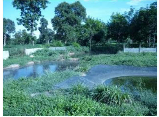
Photo 4. Ponding system. Upon removal of solid waste from the piggery floor, wastewater might be treated in a ponding system. These systems can be sophisticated and in the case shown it includes a covered subsurface flow constructed wetland (notice the rubber leaning with water accumulation on the top) and a second and third polishing pond (right upper corner), Yasothon Province, August, 2008.
