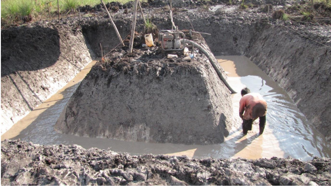
Figure 5.8: Fish pond being constructed in the NLPSF, photo by BNF
