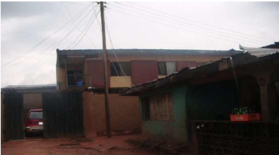
Plate 4.2: A typical haphazard and unstructured connection to the electricity grid Source: Fieldwork (2012)
