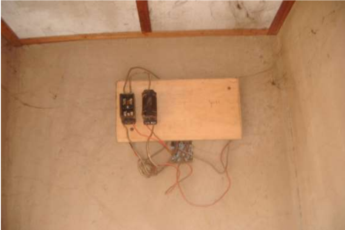
Plate 3.9: A typical household without electricity meter and on a direct connection (DC) consumption to the national grid
