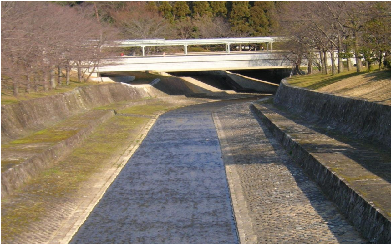
Figure.1.3. Geometry of a Compound Channel
