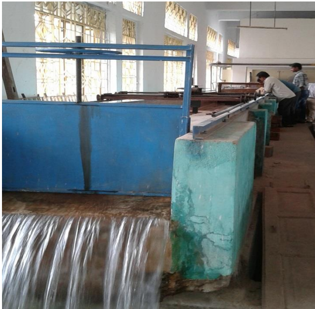
Figure 3.7. Photo of Tailgate at down stream
