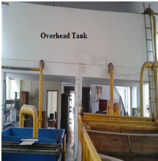
Figure 3.3. Front view of RCC Overhead Tank
