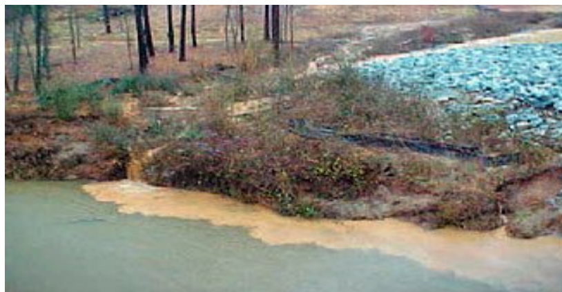
Overland runoff from disturbed areas often contain excessive sediment in addition to water. (USGS)
