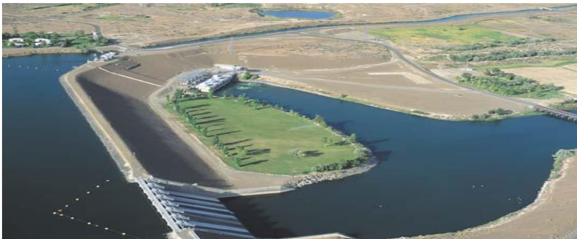
Fig 2. C.J. Strike Dam, an earth dam in Idaho
