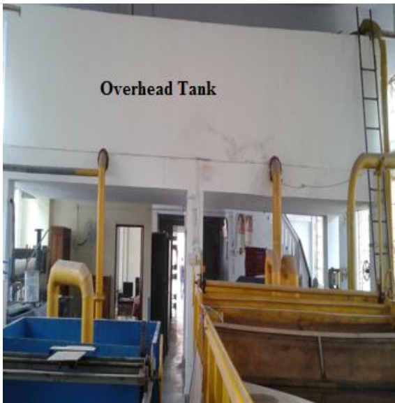
Fig 3.6 front view of overhead tank
