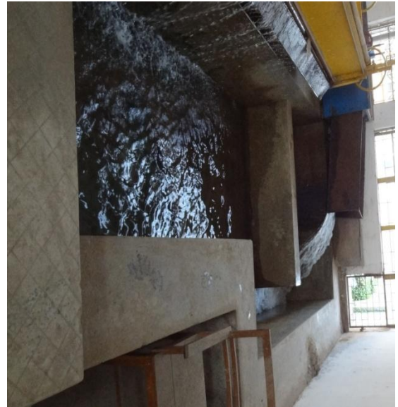
Fig 3.7 photo of volumetric tank
